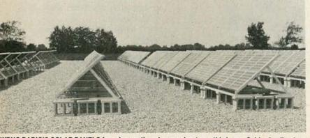
WBNO RADIO'S SOLAR PANELS face due south and cover about one-third acre. Cables leading from each panel connect to the computer-control center where the power is distributed, first to the AM transmitter, then to storage batteries. Any surplus power is used for station lighting, teletype machines, the AM console, etc.
