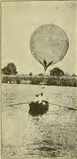
The balloon should be spherical in shape and made of some very light material of close texture. Light silk is one of the best materials for the purpose. Stitch the gores well together with strong, fine silk and coat the balloon with linseed oil varnish—a very thick coat. The neck of the balloon where
