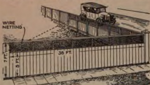
The Possibility of Accidents at a Street Crossing was Greatly Reduced by Substituting Wire Screening for Wood in the Upper Part of the Fence
