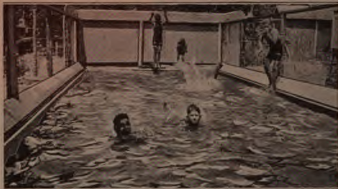
Including the Fence and a Small Bathhouse This Modern Reinforced-Concrete Swimming Pool was Built for Less than $500
