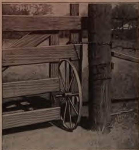
A Wheel from a Discarded Cultivator, Attached to a Farm Gate as Shown, Makes It Easy to Open and Close the Latter
