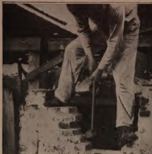
Boiler Tubes Repaired by Driving In Short Pieces of Pipe have Given Service without Trouble for Over One Year
