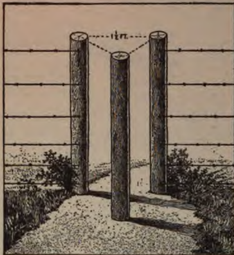
To Enable Pedestrians to Pass through a Field without Danger of Cattle Escaping, a Gate was Built of Three Posts
