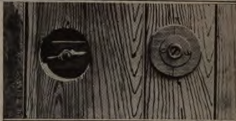
Sliding Doors Fitted with This Spring-Type Lock Provide Additional Security to Either Garage or Barn
