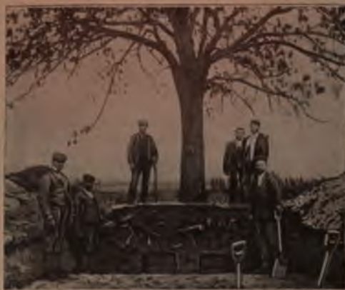
By Digging Out the Ground Properly and Providing Runways of Lumber It Is Possible to Remove Large Trees Successfully
