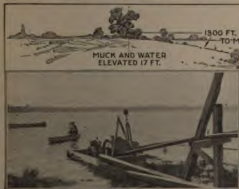
The Barge is Anchored near the Shore and Carries the Pump and Engine
