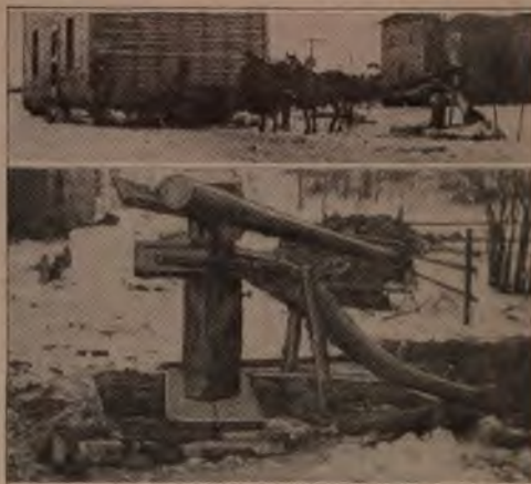
The Building was Moved Nearly One-Half Mile over Rough Ground by the Use of This Makeshift Capstan Built of a Large Tree Fork
