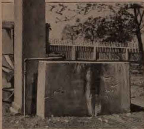
This Concrete Outdoor Farm Cooking Stove can be Made Handily with Simple Forms
