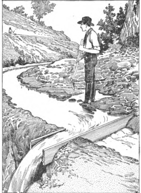
Spillways in Irrigation and Mining Ditches on Hilly Ground Prevent Washouts
