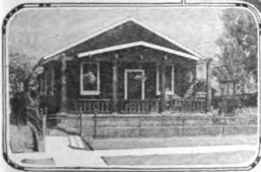
The Fence is Built Up of Pipe and Fittings, with Pickets of Heavy Wire and Attached to Short Pieces of Pipe Anchored in the Concrete Base, Either with Brimstone or Lead
