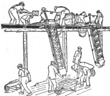
New Concrete Mixing Method
