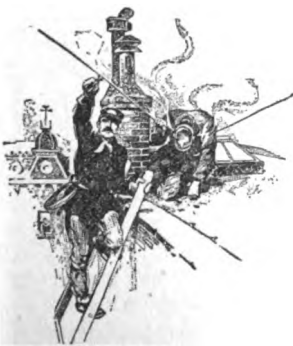
Rescuing from Contact with Live Wires.
