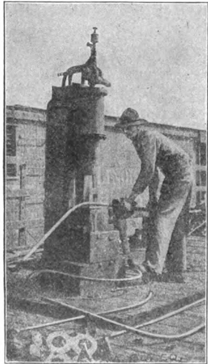
Air-Hammer for Straightening Scrap Iron.
