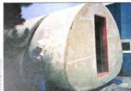
Tornado shelter is assembled from modular reinforced-concrete tube sections.
