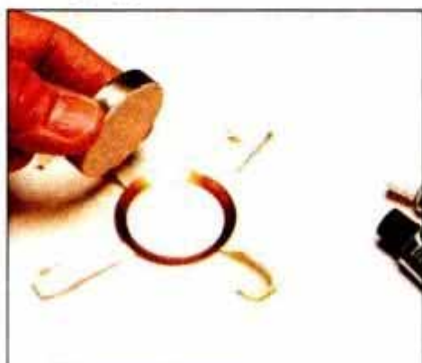
18 Seal the flange with epoxy and let it set. Then, tape the flange to the humidifier and fasten it with epoxy.
