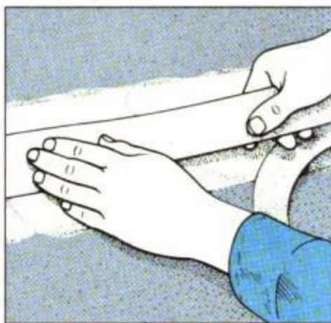
10 Once the base coat is smooth, embed the tape in the compound. Keep the middle of the tape directly over the joint line.
