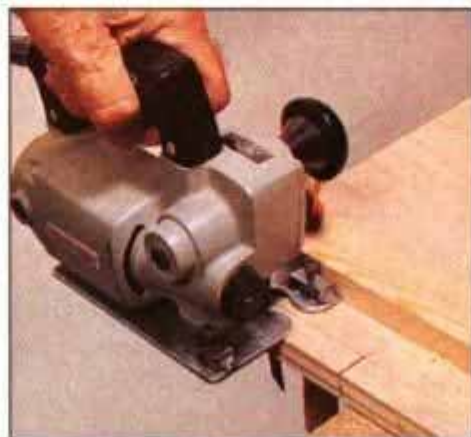
4 Cut the notch for the rear ledger on the rear upper corner of the divider. Then, apply glue and secure divider to floor.
