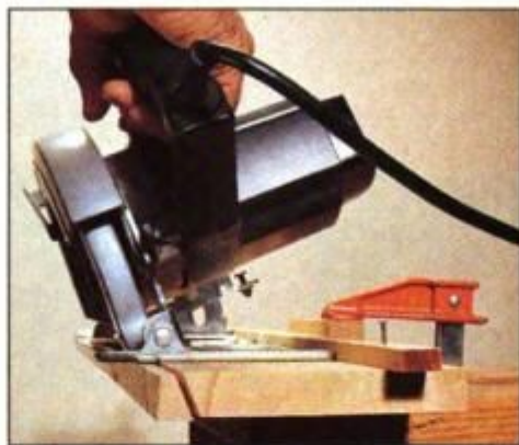
2 After planing one edge of the case sides and stiles, use a circular saw to cut 22½° bevel. Use a straight strip to guide saw.
