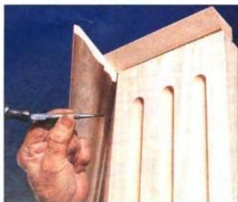
12 Attach the long crown section first. Miter the endpieces to exact length, and then glue and nail to cleat. Set nails and fill.
