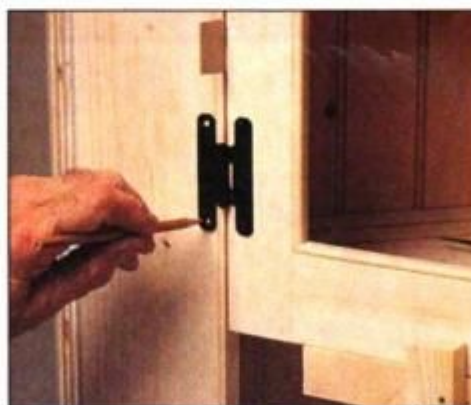
17 Clamp upper doors in place and shim to achieve equal clearance all around the frame. Then, install the H hinges.
