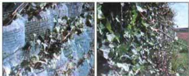
Ecowall masks old tires with vines to create noise barrier.
