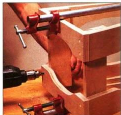
10 Use pipe clamps to hold base together while the end rails are glued and screwed. Don't glue the rear upper end rail.
