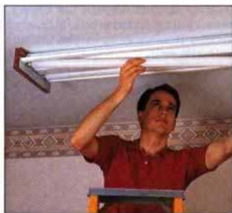
2 Rotate the lamp tubes until the socket pins are visible from below. Then, pull down carefully to remove from fixture.
