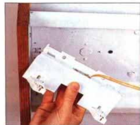
12 To remove the lamp sockets for wiring to the new ballast, simply pull inward until they clear their channel tabs.
