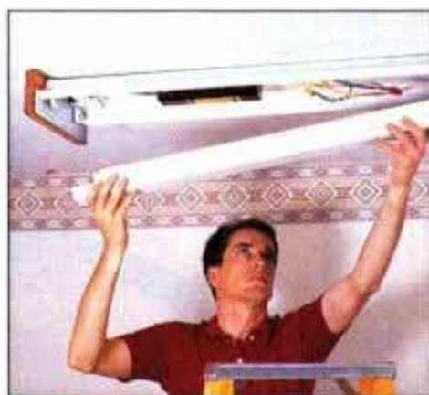
3 To access the fixture's ballast, squeeze the sides of the ballast cover to release it from the metal securing tabs.
