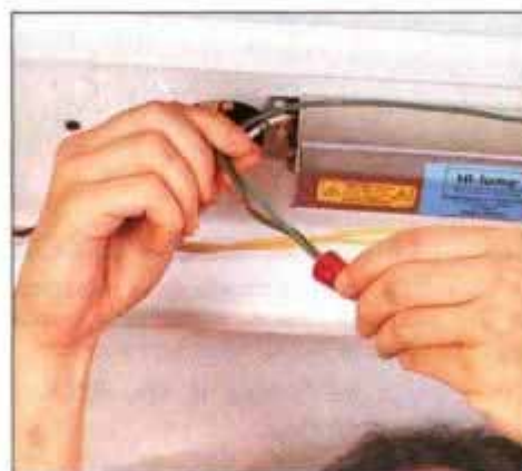
16 Use a twist connector to join the circuit ground wire to the insulated ground lead attached to the channel.
