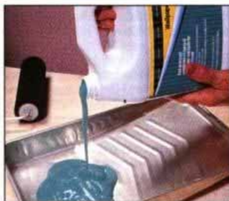
1 The thick gel formula is especially designed to cling to walls. A 1-gal. container of remover can handle about 200 sq. ft.
