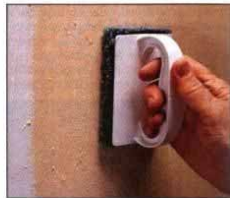
4 Remove residual paste with the woven-pad accessory that's wetted with gel. Once it's washed, the pad can be reused.
