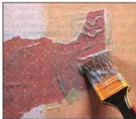
3 The 3M brush-on applicator can also be used for wall edges, baseboards, corners and trim, and for small spot applications.
