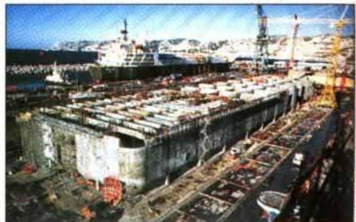
World's biggest concrete barge nears completion in dry-dock.
