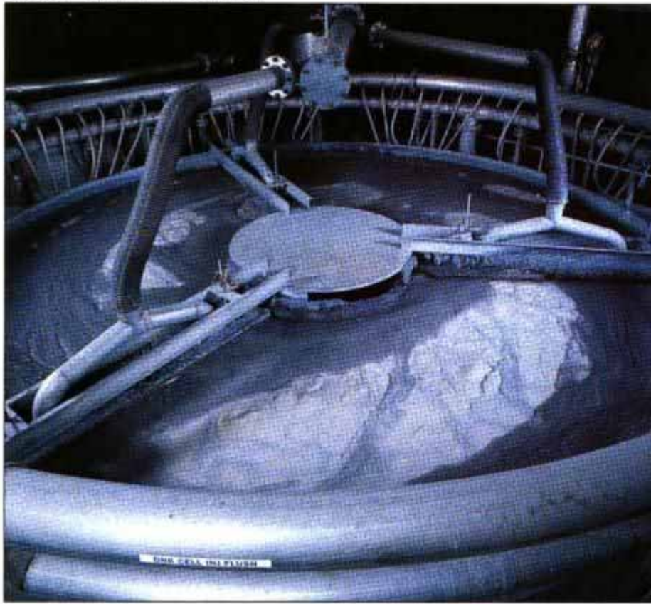
In flotation de-inking vat, vacuum tubes remove bubbles coated with ink and clay.
