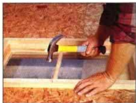
4 After sheathing, cut window opening and use 10d galvanized casing nails to secure the window to the wall.
