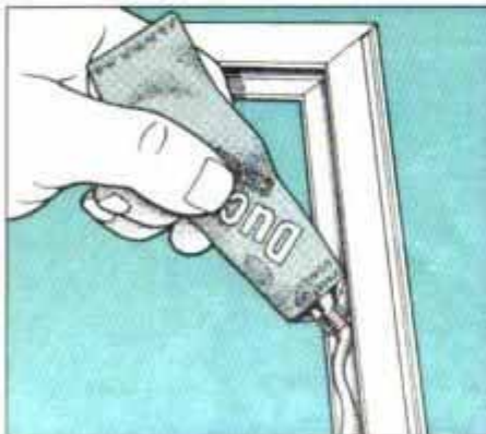
27 Apply a thin bead of cement around the ledge of the window frame. Then, lay the glass in place and press to seat.
