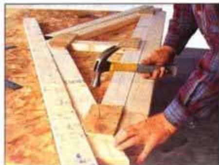
7 Build a roof truss jig on a plywood platform. Then, nail and glue ½-in.-plywood gussets to the truss components.
