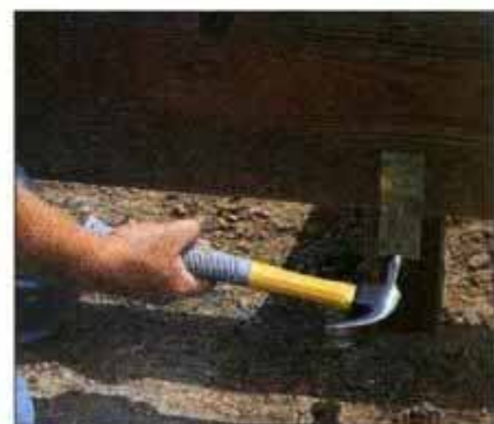
6 Anchor the footing bracket to the post with nails and the post to the double rim joist with 2 × 5 galvanized truss plates.
