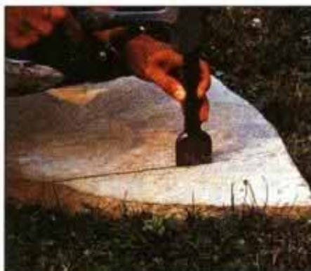
10 To cut a stone, position it on a flat piece of ground and score the cutline with a mason's chisel. Score the bottom, too.
