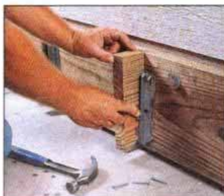
4 Lay out the joist positions, then use a scrap of 2 × 10 joist to align each joist hanger. Use proper nails to install brackets.
