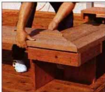
14 Bring the mitered bench sections together at the corners and screw them in place on top of the box supports.
