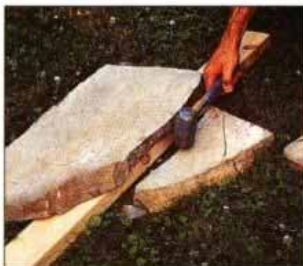
11 Once scored, place the stone over a 2 x 4 block, with the waste area unsupported. Then strike it with a hammer.
