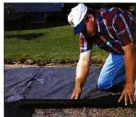
3 Remove the sod, then cover the soil beneath the deck with landscape fabric. This keeps the weeds from growing.
