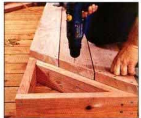
12 Set the corner boxes in position and measure for the seat planks. Prebore the ends and screw the planks to the boxes.
