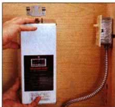
8 Screw the hot water dispenser's mounting bracket to the cabinet wall and hang the tank on the bracket.
