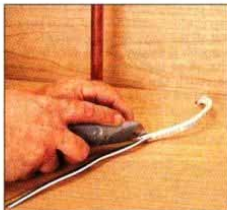
2 Strip about 10 in. of sheathing from the cable. Then strip 1/8 in. of insulation from the end of each wire.
