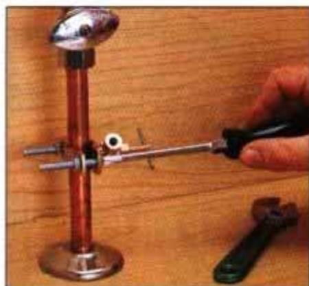
7 Mount the self-piercing saddle valve on the cold water riser pipe by drawing up the saddle bolts evenly.
