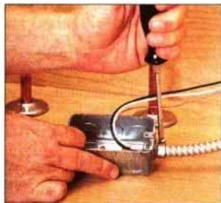
3 Feed the wires through the flexible conduit and connect the conduit to a metal duplex box with a box connector.
