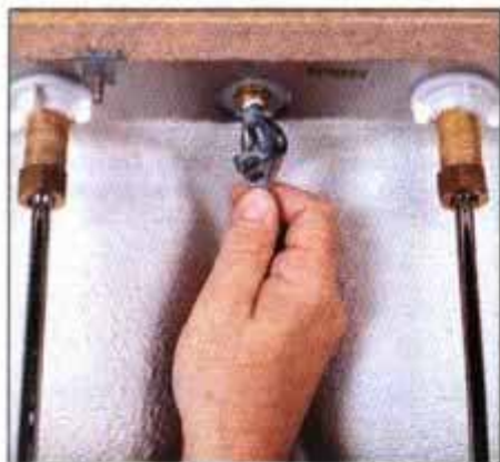
10 To seal the faucet port, wrap Teflon tape around a 1/8-in. threaded plug and then tighten it into the faucet port.
