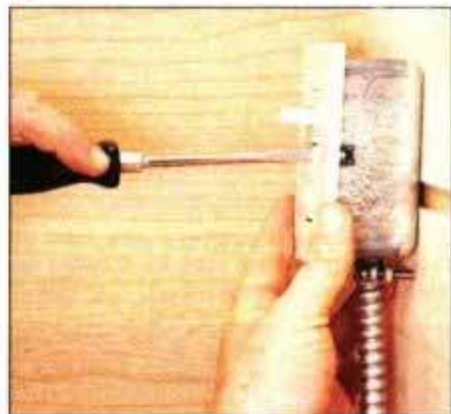
6 Install the switched receptacle in the box and fasten the cover plate. Do not plug in the unit until it's charged with water.
