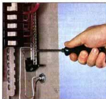
17 With main switch off, secure the white and bare wires under terminal lugs on the neutral/grounding bus. Tighten firmly.
