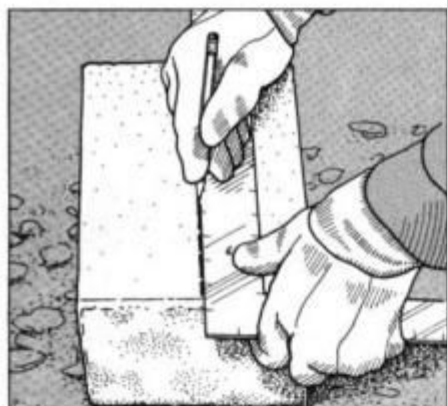
16 Draw the centerline around the block using a pencil and framing square. For the best results, accuracy is important.
