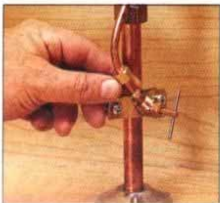
13 To connect the water supply, slide the saddle valve's compression nut and ferrule onto the supply tube. Lubricate and tighten.
