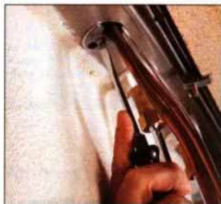
12 Use the factory-installed fastening screw and mounting washer to fix the water-heater faucet in the hole from below.
