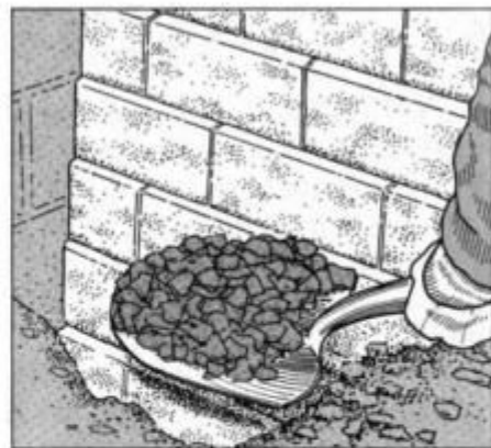
19 Once blocks are installed, lock the first two courses in place by filling the trench in front and back with crushed stone.
