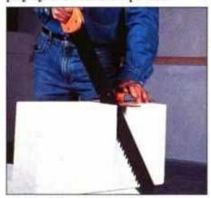
The blocks can be sawed to length with a crosscut saw from the manufacturer. They're finished with stucco or thin-set tile.
