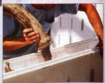
**2** When the blocks are built up to a sufficient height, they are braced with framing lumber. Next, concrete is pumped into the forms, and when the concrete hardens, the braces are removed.
