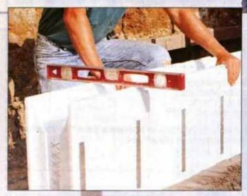
1 The first row of polystyrene blocks is set into a wet concrete footing or on top of dry concrete. The forms are set level and plumb. Subsequent forms snap onto the top of the first row.
