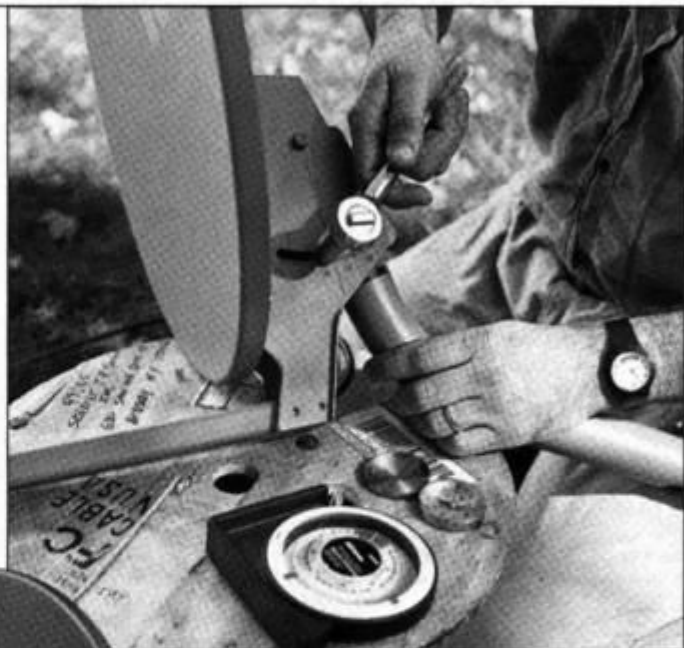
LNB angle is secured after proper elevation is obtained by entering your ZIP code in DSS receiver.
