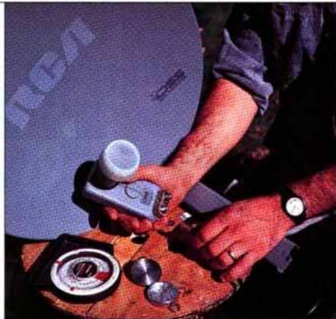
Coaxial cable is fed through support arm and connected prior to securing LNB (low-noise block) converter to arm.
