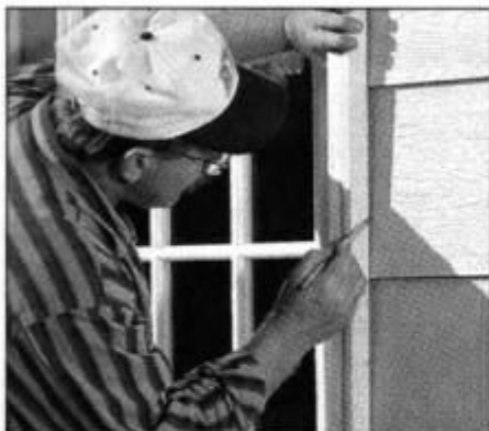
11 Set the door in place with the molding against the siding. Then, trace the molding perimeter on the siding.
