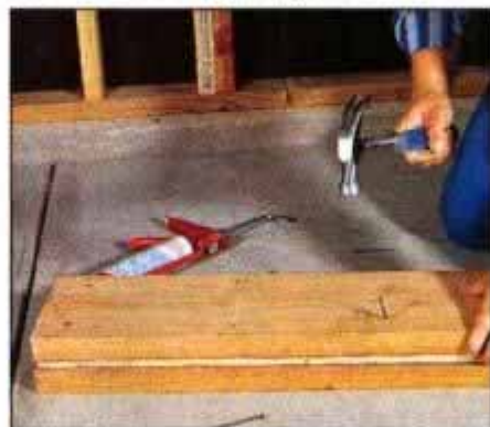
3 Sandwich the piece of plywood between the 2 x 8s and nail through from both sides. Use eight 16d nails on each side.
