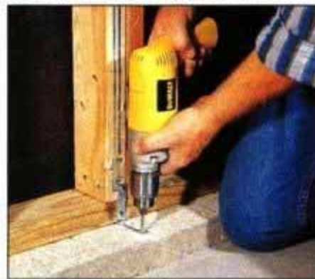
7 In a garage installation like ours, use an L-bracket to secure soleplate to floor at opening. Otherwise, nail to floor.
