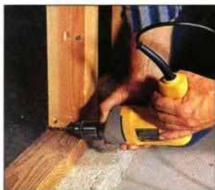
8 To locate opening on the outside of the house, bore 1/4-in. holes through the wall from the inside at the opening corners.
