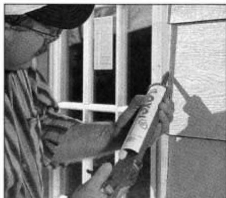
17 Seal the door against the weather with a bead of high-quality flexible caulk applied around the casing perimeter.
