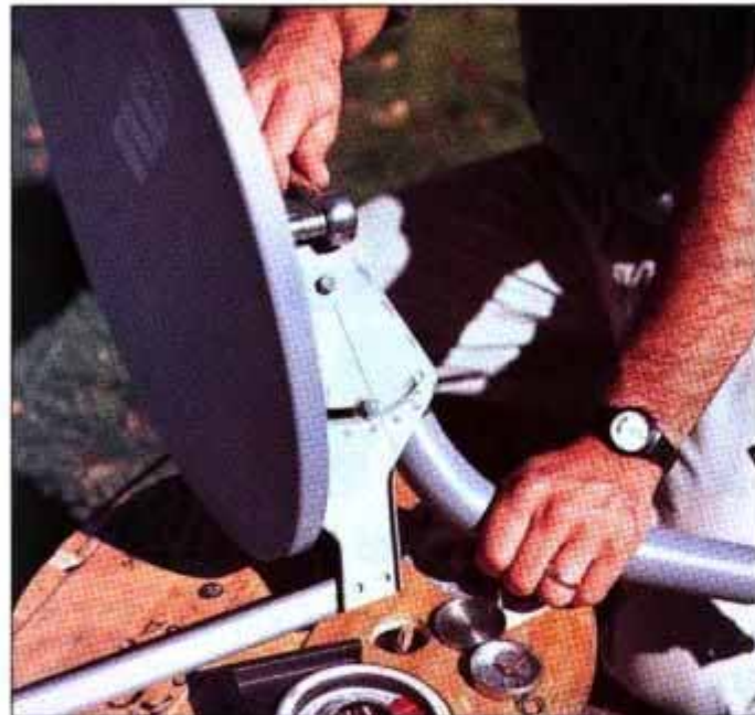
In the pre-installation assembly, four flat head bolts with self-locking nuts secure the dish to the support arm.
