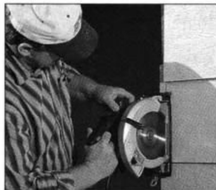
12 Use a circular saw to trim the siding. Set the saw for a 1/4-in.-deep cut, or just enough to go through the siding.
