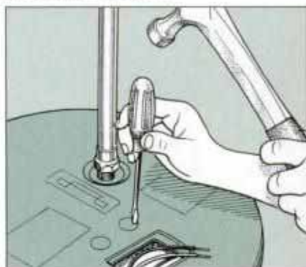
21 Locate a knockout on the top of the tank and force it down with a screwdriver and hammer. Break it off with pliers.
