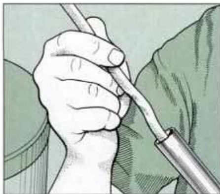
23 Cut a piece of conduit to length and slide it over one end of the electrical circuit cable. Avoid damaging the insulation.
