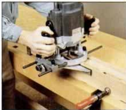
7 Cut the slat mortises in the side rails using a plunge router. Again, clamp two rails together to support the plunge router.
