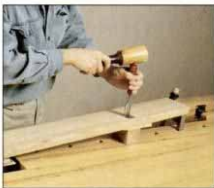
9 Fasten an arm to the workbench, and support it at a slope. Cut the through mortise for the leg tenon using a chisel.
