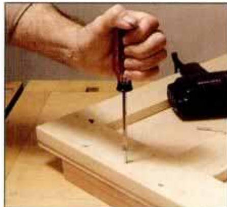
1 After assembling the jig base, use glue and screws to attach the guide rail support blocks to both ends of the base.
