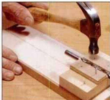
1 Align bit squarely on temporary bit-support block and tack cleats on each side of bit. Bit is aligned with base centerline.
