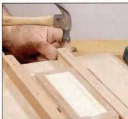
13 Tack rabbeted carriage guides to tilting platform and check for alignment. Then, secure guides with screws.
