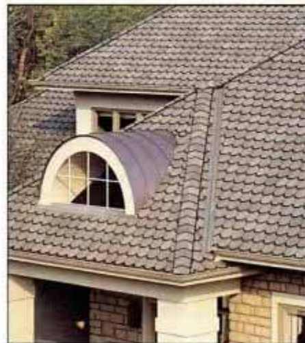
Architectural asphalt shingles are thick and have shadow lines like red tile (top) or like slate (above). They come in a range of colors, including blue and green.
