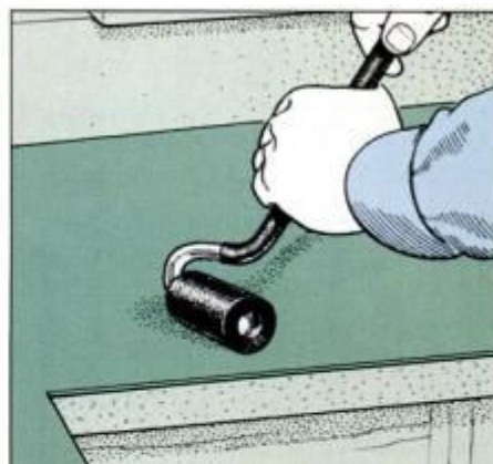
12 Roll the entire surface, to ensure a good bond with the old counter, using a rubber J-roller or pastry rolling pin.
