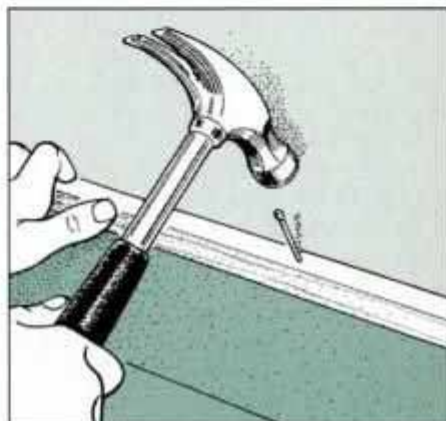
20 Cut strips of hardwood to size for use as backsplash caps. Then bore pilot holes and attach the caps with 8d finishing nails.
