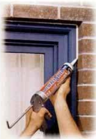
USE IT AROUND DOOR JAMBS. AROUND WINDOW FRAMES. ANYWHERE YOUR HOME LOSES ENERGY.
