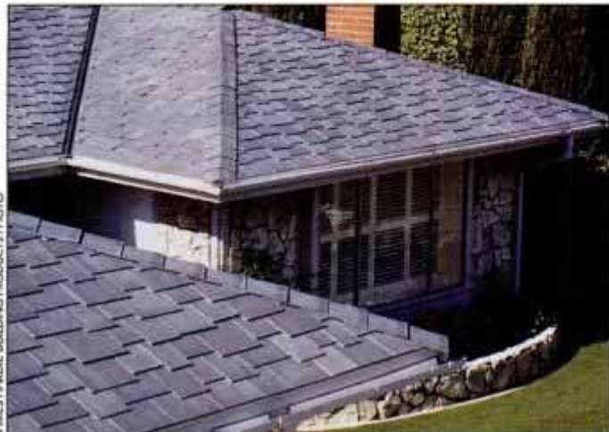
Fiber-cement tiles offer the look and color of slate while providing comparable durability and fire retardance.
