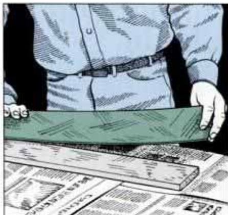
17 Apply laminate to strips of 1/4-in.-thick hardboard to create the new backsplash. Trim the edges flush with a router.
