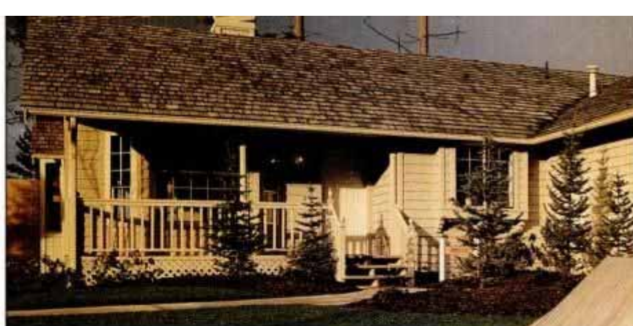
CEDAR SHAKE & SHINGLE BUREAU PHOTOS
