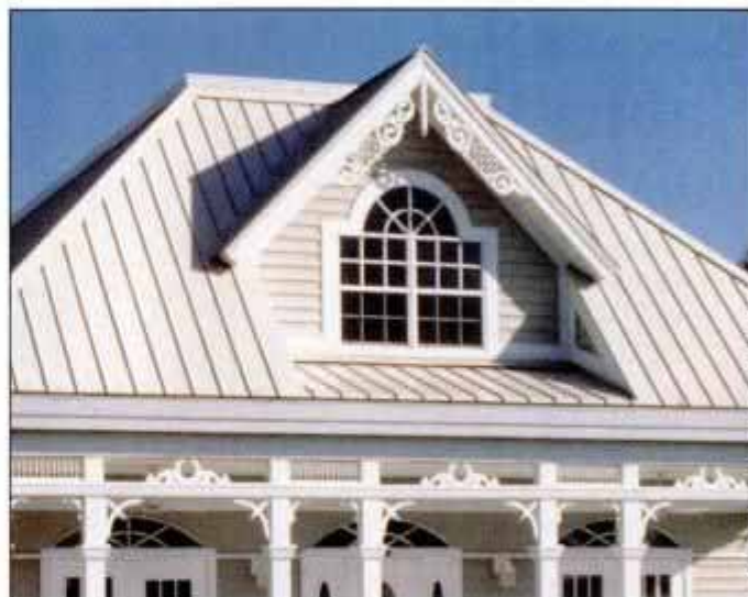
Standing-seam steel roofing is available in a range of colors, including gray, green, blue and red. It can be factory-coated so it won't need to be painted, or it can be unpainted.
