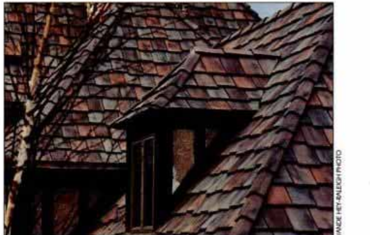
Concrete roof tile looks like slate, and uses aggregate instead of fibers to add strength. It comes in a variety of colors and patterns.
