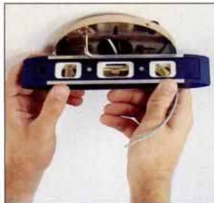
8 Use a small level to check that the plate is level in both directions. Tighten the screws into the brace to adjust the plate.
