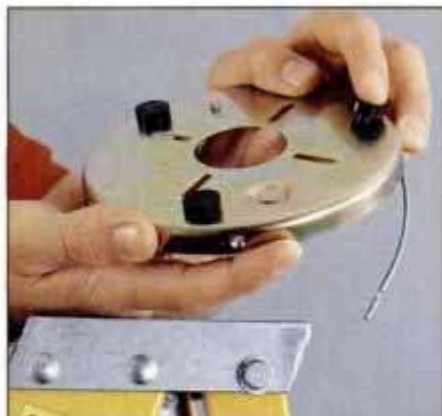
6 The fan that we installed has three rubber vibration-absorbing pads that fit in holes in the fan mounting plate.
