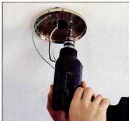
7 Drive screws through the mounting plate and box, and into the 2 x 4 brace until the plate rests against the ceiling.
