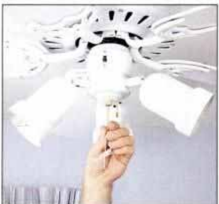
18 Set pull-chain switches so the light is on and the fan is off. Wall switch will control light while pull chain controls fan.
