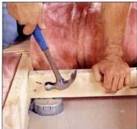
4 Install a 2 × 4 brace to support the weight of the fan. If you don't have attic access, use a retrofit fan box kit.
