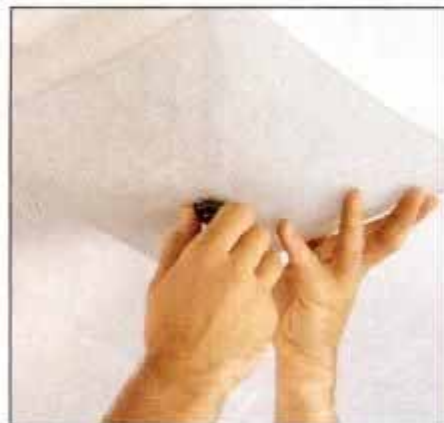
1 Shut off the circuit that powers the old ceiling fixture, and remove the lamp's diffuser to access the mounting plate.
