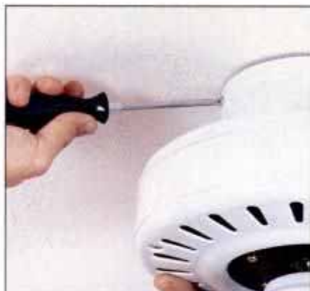
12 Hold the assembly in place on the mounting plate. Add the third mounting plate screw and tighten all firmly.
