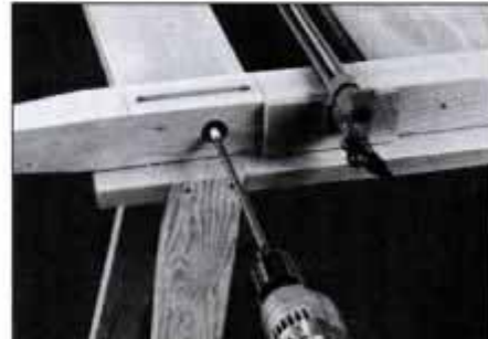
11 Use a long bit to bore slowly through the post holes and into the headboard and rail tenons.
