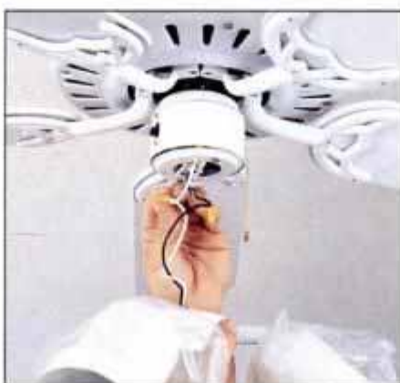
16 Lift the light kit and join the white leads with a wire connector. Then join the kit's black lead to the remaining lead.
