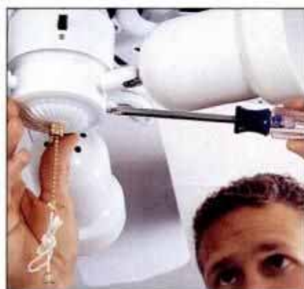
17 Screw the light kit to the switch housing and install the bottom cap, which contains the light's pull-chain switch.
