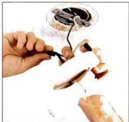
2 After removing the screws that hold the fixture mounting plate in place, twist off the wire connectors and set the unit aside.
