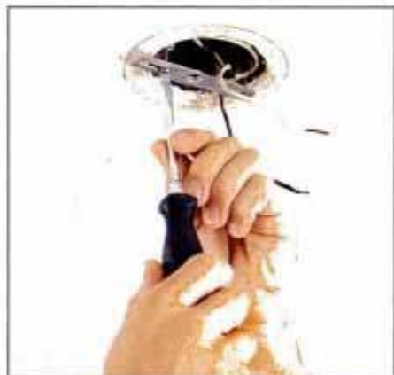
3 If the mounting plate was secured by a threaded nipple, remove the mounting bracket from the fixture box.
