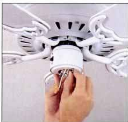
15 Using the same screws and tapped holes, install the light kit adapter ring on the bottom of the switch housing.
