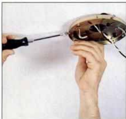
9 With mounting plate firmly attached, install two of the three screws in the plate side for holding the motor assembly.
