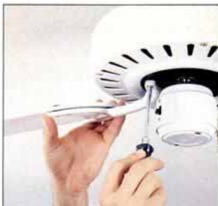
13 After mounting the blades on their metal brackets, screw each bracket in its place on the motor assembly.
