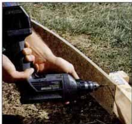
6 Notch the end of the 2 × 4 form where the curved section will meet it. Screw the curved hardboard form to the notch.
