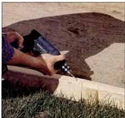
4 Join form lumber end to end by driving a deck screw through the edge of one piece and into the end of another.
