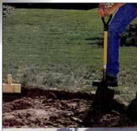
1 Begin the sidewalk installation by stripping the sod from the form area. Dig a trench just deep enough for the forms.
