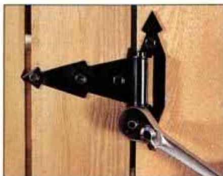
14 Use a socket wrench to drive lagbolts that secure the gate hinges. Bore pilot holes for the lagbolts.
