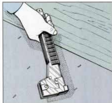
1 Begin siding job by installing builder's paper at the bottom of the wall over the sheathing. Staple paper every 8 to 12 in.
