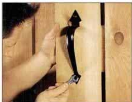
16 Gate hardware usually comes with the necessary screws or bolts. Install the gate handle and then check gate operation.
