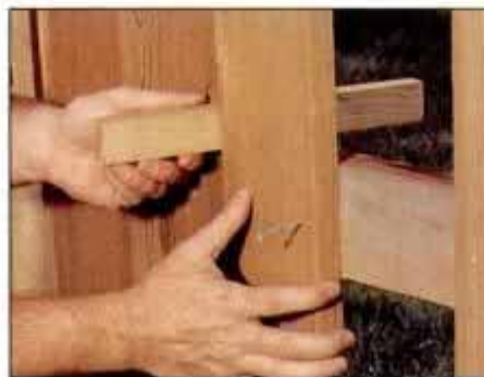
11 After nailing a slat to the top rail, position the slat bottom with the spacer strip. Drive two nails at each location.
