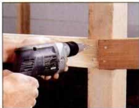
7 After cutting the rails to exact length, set them in the post notches and secure them with 3-in.-long deck screws.
