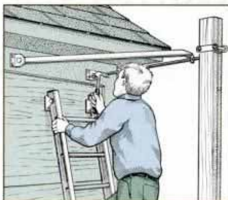
Slide the pump mechanism and top braces over the pole. Then stand the pole in place and nail the top braces to the house.
