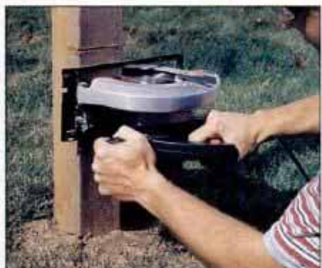
5 Set the blade depth on your circular saw to the thickness of the rails, and make a series of cuts in the notch waste area.
