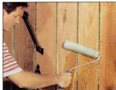
18 Apply sealer to fence with a roller, brush or garden sprayer. Then, apply a UV-screen sealer to prevent weathering.
