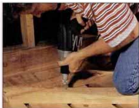
13 After the horizontal gate crossmembers are in place, check that the gate is square and secure a diagonal brace.
