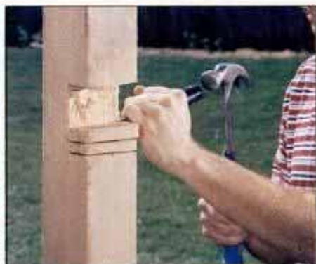
6 Use a sharp chisel to remove the waste from the notch area. Then, test fit the rails and adjust the notch if necessary.
