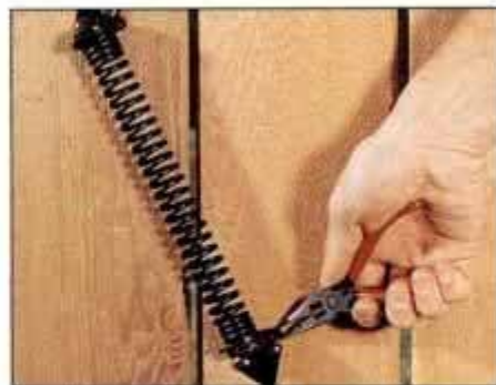
15 After installing the gate spring, adjust the tension by removing a pin, turning a hexhead nut and reinstalling the pin.
