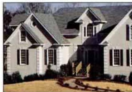
Modern acrylic stucco systems look like traditional portland cement versions, but better resist hairline cracking.
