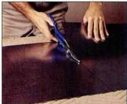
11 Use a felt marker and straightedge to lay out cut and bend lines on sheetmetal. Make cuts with heavy-duty shears.
