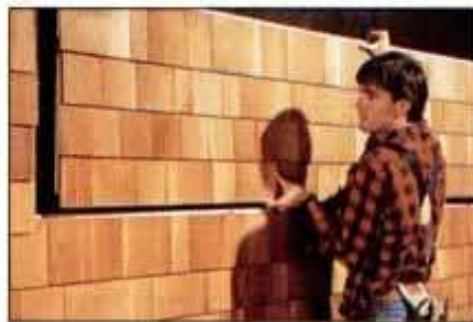
Cedar bevel siding (far left) and shingles (above) are durable and attractive. Shingles can be individually installed (above) or panelized (left). Any cedar siding is durable, but it requires paint, stain or sealer.
