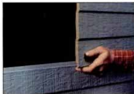
Hardboard siding comes in individual pieces or panels. It may be primed or have a factory-applied topcoat.
