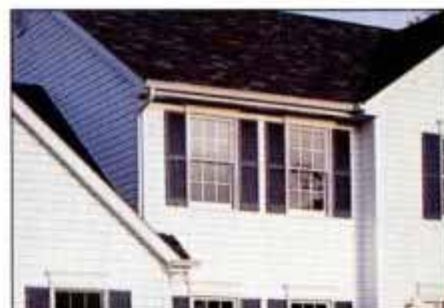
After 40 years, aluminum siding is still popular. Often it's installed with new aluminum gutters, soffits and trim.
