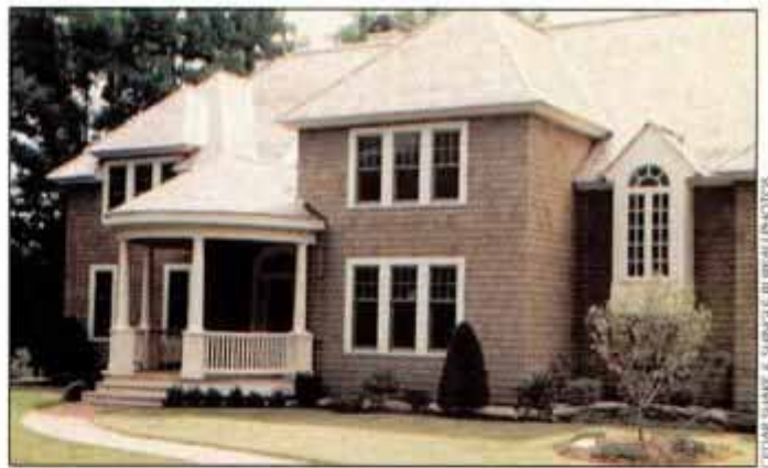
Cedar bevel siding (far left) and shingles (above) are durable and attractive. Shingles can be individually installed (above) or panelized (left). Any cedar siding is durable, but it requires paint, stain or sealer.
