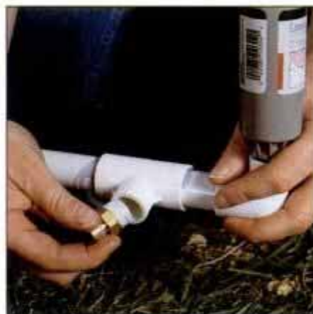
6 Thread pressure-activated brass drain fittings into horizontal drain tees. Use Teflon tape to seal threads and tighten securely.
