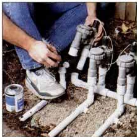
8 Use threaded male adapters and glue to join the piping to the zone-control valves. Each valve controls one sprinkler branch.
