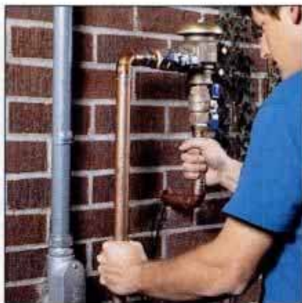
12 After assembling vacuum breaker with pipe and fittings, slide assembly through hole. Vacuum breaker remains vertical.
