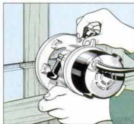
16 Place a router on the straightedge guide and cut the cable groove through the foam panels and furring strips.
