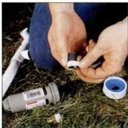
5 Make final threaded connections with Teflon tape to ensure leakproof joints. Be sure to orient directional heads correctly.
