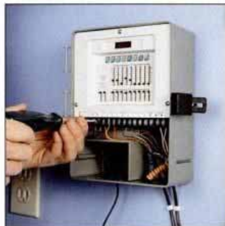
16 Mount the electronic control panel and connect the cable wires from the zone valves to the terminals in the panel.
