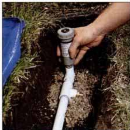
7 Place coarse gravel under drain fittings to help keep soil from clogging fittings. When backfilling, also add gravel on top.
