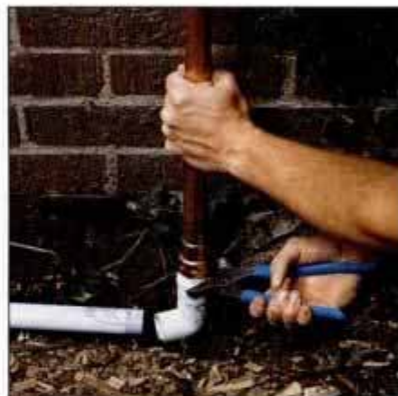
13 After gluing a PVC threaded adapter to 90° fitting, connect to copper feed line. Then, glue PVC supply pipe to fitting.
