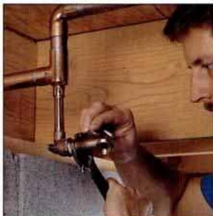
15 Before connecting inside piping to outside piping, install a reducing tee and boiler drain so the pipes can be drained.
