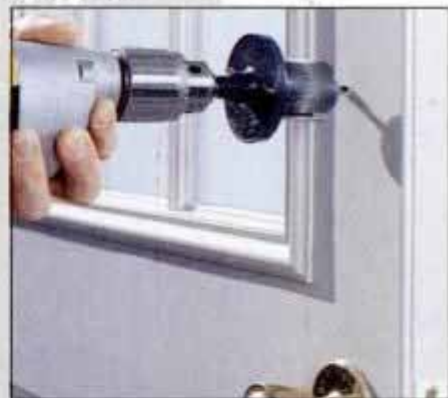
3 Remove the holesaw and slide it into the pilot hole on the other side of the door. Finish the cut from this side.
