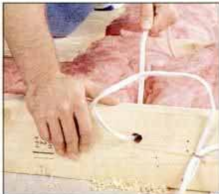
5 When crossing ceiling joists, bore a cable hole through the center of the joists and pull the cable through.
