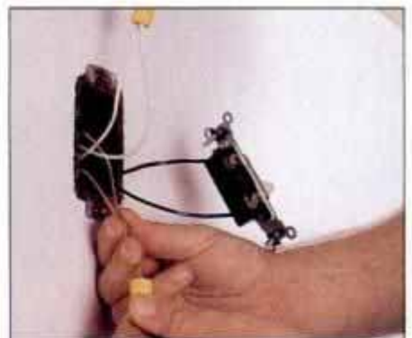
14 Join the wires to the back of the switch, then press the switch into the box. Install a cover plate and test.
