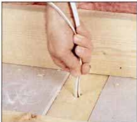
4 Feed two cables—one for the switch, and one for the floodlight—through the switch box hole and into the wall cavity.
