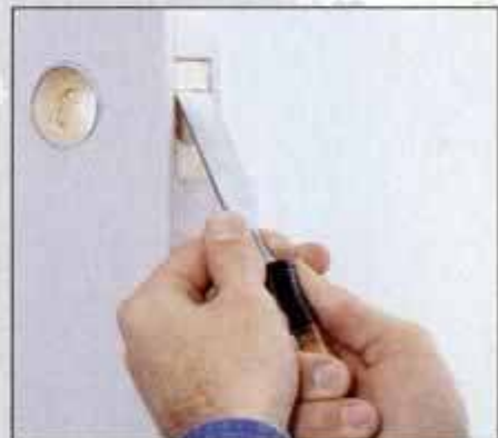
6 Remove the bolt assembly, then chisel out the stock below the plate (about \frac{1}{8} in.) so the bolt plate fits flush.
