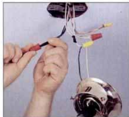
15 To access power, join all white, black and ground wires. Then join the black fixture wire to the white switch wire.
