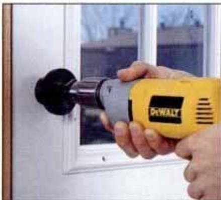
2 Use a holesaw to bore a hole for the lock bolt. Stop when the pilot bit breaks through the other side.
