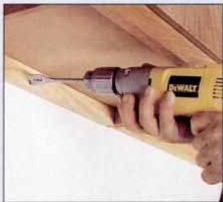
1 Locate the best position for the electrical cable, then bore a hole through the rear cabinet rail and into the wall.
