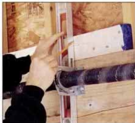
9 Establish and mark the centerline of the door, then transfer this mark to the bracket support board above the door.
