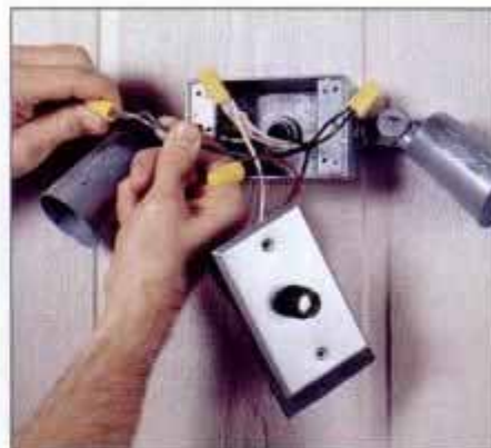
9 Join all white wires together and all ground wires together. Then hook the black (hot) wires to the photocell.
