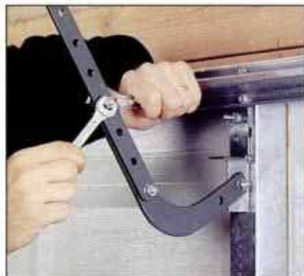
13 Attach the bar link to the door and traveler with keyed pins. Then bolt the two halves of the link together.
