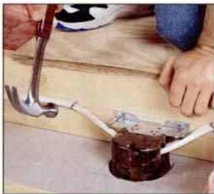
2 Staple the new cable alongside the ceiling joist within 8 in. of the ceiling box and every 4 ft. thereafter.
