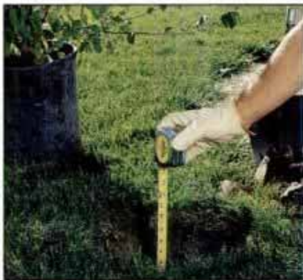
1 Dig the hole slightly larger and deeper than the nursery pot and check all measurements with a tape measure.
