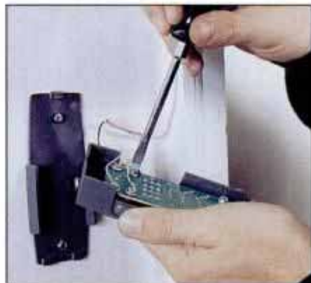
17 Screw the base of the control to a garage wall and tighten each color-coded wire to the control's terminal block.
