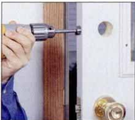
4 Bore the hole in the edge of the door, making sure the bit is perpendicular to the door in both directions.
