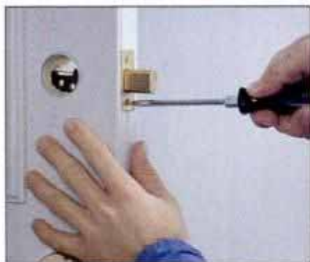
7 Slide the bolt assembly into place again. Then bore pilot holes and attach the assembly with the screws provided.
