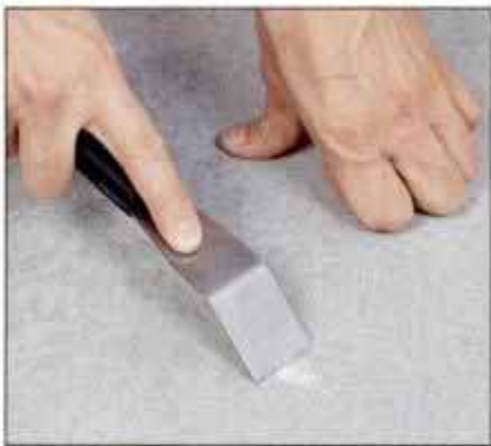
1 Use a putty knife to scrape any paint splatters, construction adhesive or other debris from the surface of the floor.
