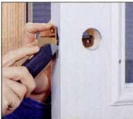
5 Slide the bolt assembly completely into its hole, then scribe around the bolt plate with a sharp utility knife.
