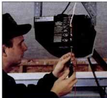
18 Make the necessary performance adjustments by turning the screws located at the back and bottom of the power unit.
