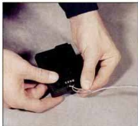
14 Insert the low-voltage wires into the receiver/sender-terminal slots and tighten with a small screwdriver.
