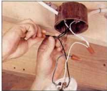
7 To get power from a ceiling fixture, join the like-colored wires from the new cable to those of the power feed in the box.
