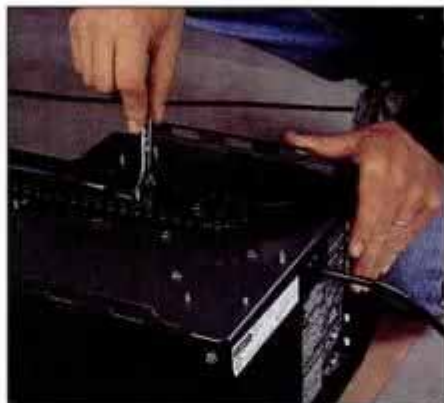
8 After connecting the return end to the traveler, tighten the chain by adjusting the bolt on the power unit.
