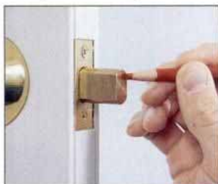
10 Mark the face of the deadbolt with a grease pencil. Then throw the bolt against the jamb to mark the jamb hole.
