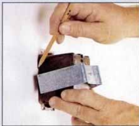
3 Position a cut-in switch box at the same height as other switch boxes in the room. Then trace around the box.
