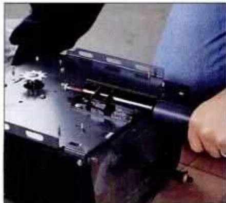
4 Carefully slide the capped end of the track tube into the bracket that's mounted on top of the power unit.
