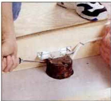
1 To access power from an existing ceiling box, first use a screwdriver to punch a new box hole for the supply cable.
