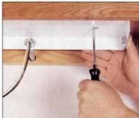
10 Once the cable is fed through the conduit, attach the fixture channels directly to the bottom of the cabinet.
