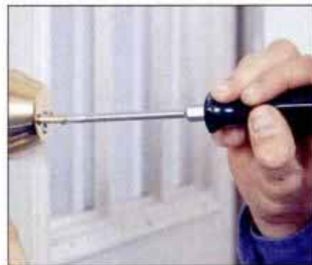
9 Securely join the two sides of the lock mechanism by driving two screws through the inside lock mechanism.
