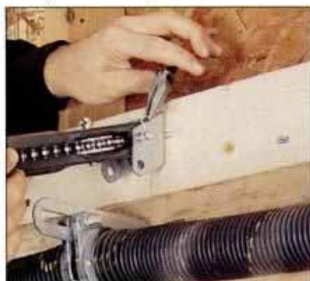
10 Attach the support bracket to the brace with lag screws and lock the idler into the bracket with a keyed pin.
