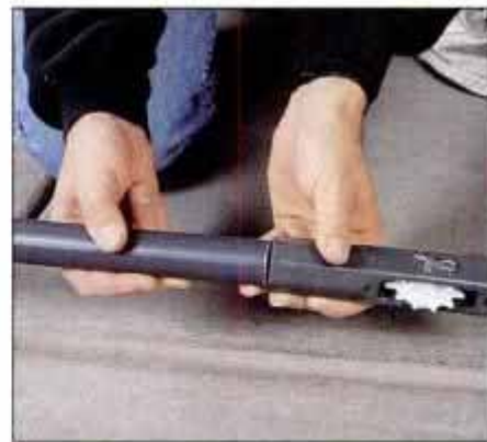
3 Slide the idler assembly onto the door end of the tube. The idler will later fit into a header bracket.
