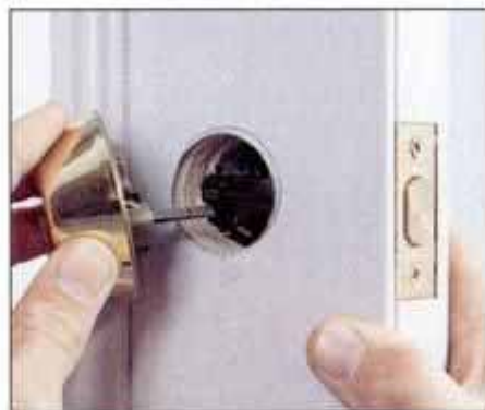
8 Slide one side of the lock mechanism through the slot in the bolt assembly. Then slide the other side into place.
