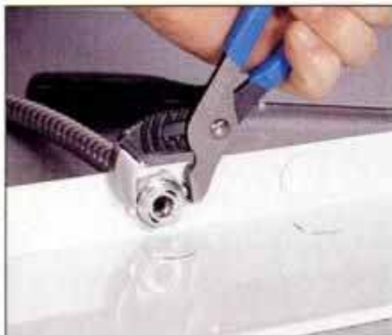
9 Protect exposed cable lengths with flexible conduit. Join the conduit to the fixtures with box connectors.
