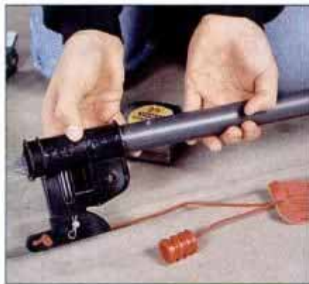
2 Slide the traveler assembly onto the end of the track tube and position it 39 to 41 in. from the power unit.
