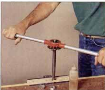
13 Cut the threads on the axle. Take small turns, back off and then cut some more. Use plenty of cutting oil.
