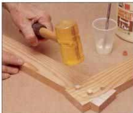
8 For added strength, pin end-lap joint with dowels after applying glue. When glue has set, trim ends flush.
