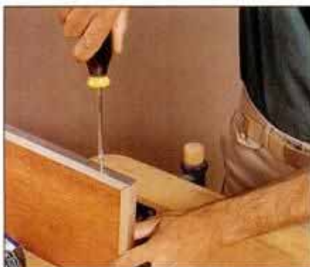
7 Screw the channels in place using self-tapping round head screws. These screws hold firmly in marine plywood.
