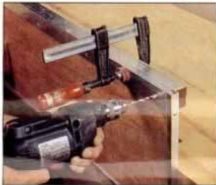
9 Clamp a scrap block and an angle to a side panel. Bore pilot holes through the panel, the angle stock and the channel.
