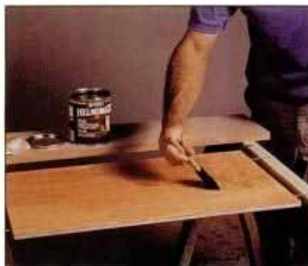
2 Suspend the panels from between sawhorses. Apply the exterior polyurethane finish on the panels' faces and edges.
