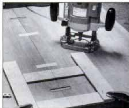
15 While cutting the hinge mortises, guide the router with a simple frame. Clamp and tack nail the frame in place.
