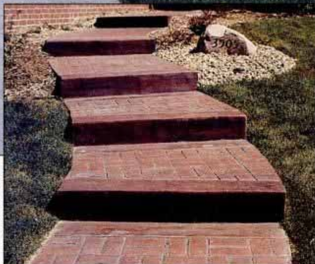
Concrete can look like stone, slate or brick. At this house, it was finished to look like stone on the drive and brick on the walkway. Even the "wood beam" risers are really concrete.
