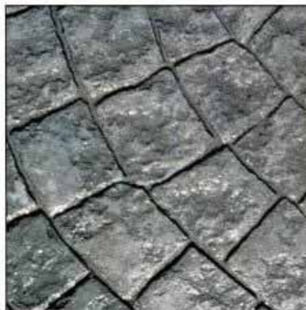
These faux granite cobblestones are finished with a sealer to give them a soft sheen and better resistance to stains.
