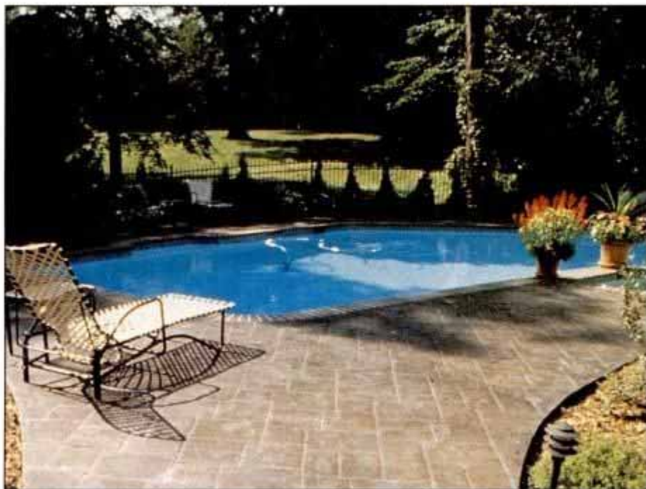
Faux-finished concrete is a good choice for a pool deck, since it wraps neatly around any shape. The pavement, including the faux mortar joints, can be colored to match or offset the pool itself and its surroundings.
