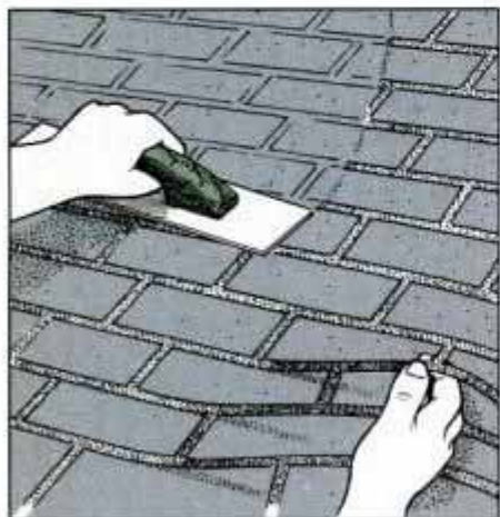
1 A stencil is laid on the wet concrete and then pressed into the surface with a magnesium hand float.
