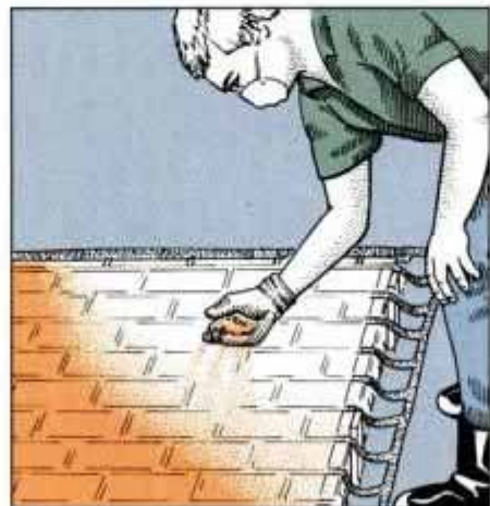
2 Colored granules, known as dry-shake compound, are spread over the stencil. The compound is worked in with a float.
