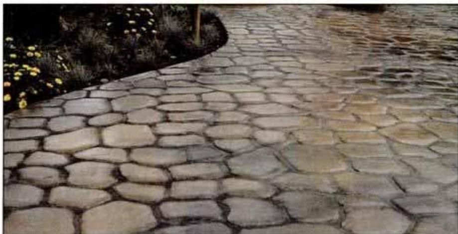
Faux-finished concrete runs the gamut in terms of its level of finish. This rustic walkway looks like smooth-surface river rock with wide dark mortar joints. The rock can be a single color, or two colors can be mingled.
