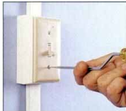
15 After the switch is wired, secure it to the extension box with screws and attach the switch coverplate.
