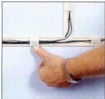
7 Lay the wires into the channel and use wire clips to hold them in place. Use wires of the same size as the original circuit.
