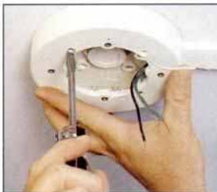
16 Fasten the ceiling box extension to its baseplate with screws before connecting the wires to the ceiling fixture.
