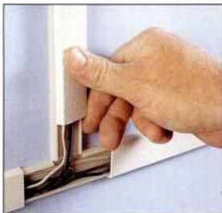
8 With wires in place, measure the trim channels exactly and snap them in place over the base channels to conceal wiring.
