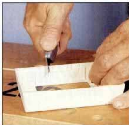
11 Use a utility knife to cut the ends of knockouts in the extension boxes. Then break away the knockouts with pliers.
