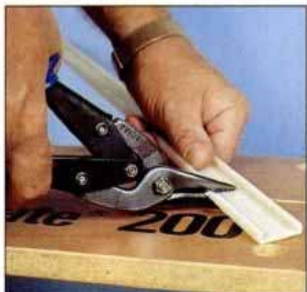
3 Use tin snips or a hacksaw to cut the base channel to length. Use a hacksaw only when cutting the trim channel.
