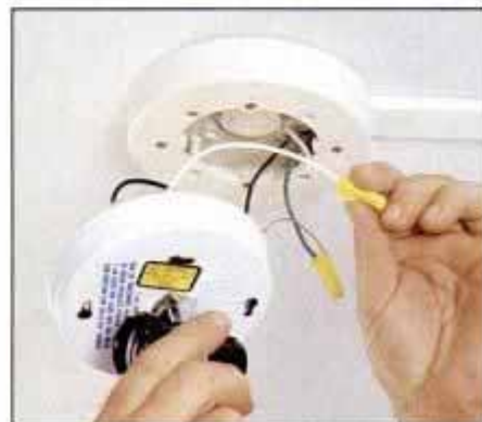
17 To wire the ceiling fixture, join all like-color wires with twist connectors. Then, install the bulb and diffuser.
