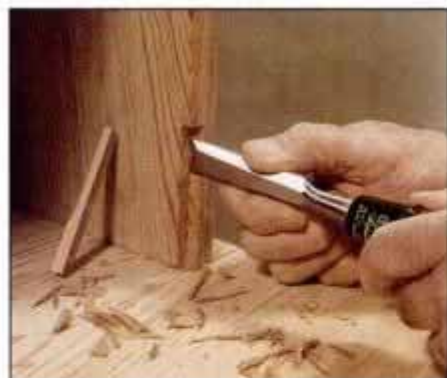
10 Use a sharp chisel to remove the worn section. Pare the sides of the notch smooth and flat so the patch seats well.
