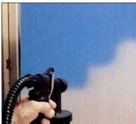
6 For even coverage, overlap each pass about 50%. Start each pass so pattern is centered on bottom edge of the last pass.
