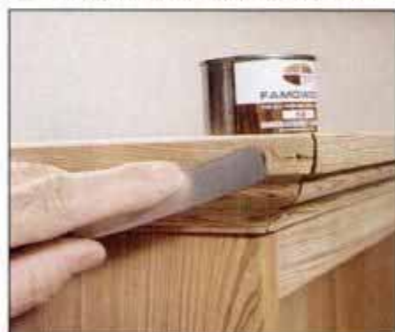
12 Fill nail holes and small cracks with wood filler. Apply the filler with a small putty knife and sand it flush when dry.
