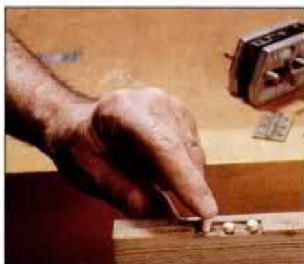
18 Use dowels to plug worn screw pilot holes. A doweling jig will yield the most accurate holes for dowels.
