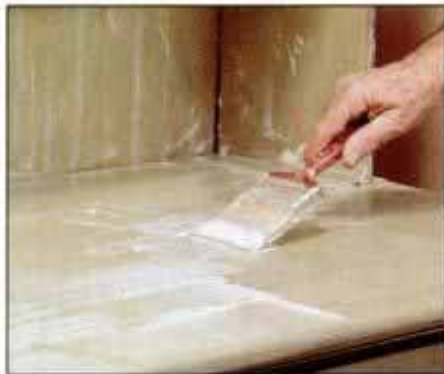
4 Apply the stripper with a soft brush. Avoid overbrushing water-base stripper. Let stand until paint is soft.
