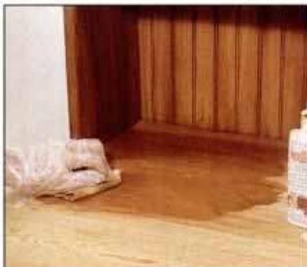
20 Use a cloth to apply gel stain. If the application is too light, apply a second coat. If too dark, wipe with mineral spirits.
