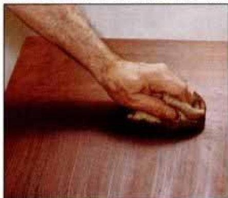
13 After the wet look of the filler is gone, wipe away the excess with a burlap cloth. This leaves filler packed in pores.
