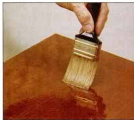
16 Then, remove all excess varnish from brush and gently wipe the wet coat with the bristle tips in the direction of the grain.
