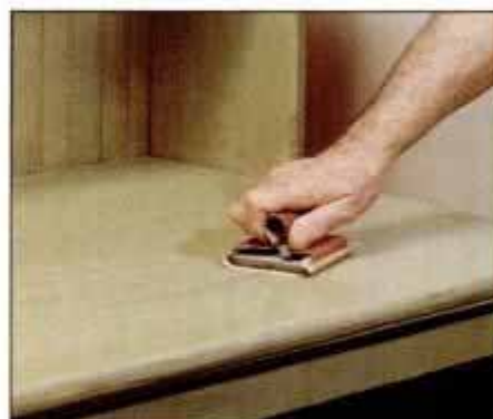
3 Lightly sand the old finish with 150-grit paper before stripping. The scuffed surface makes the stripper more effective.
