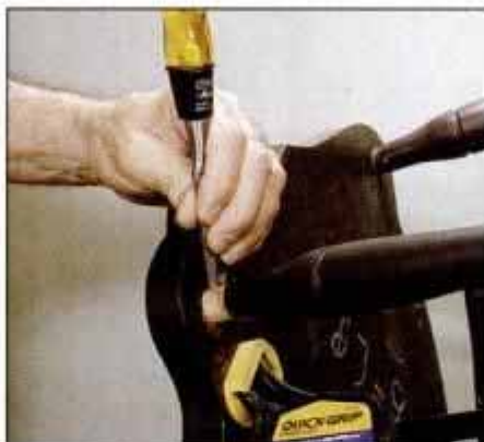
1 After spreading apart the loose joints, prepare for gluing by using a chisel and file to clean off all the old glue.
