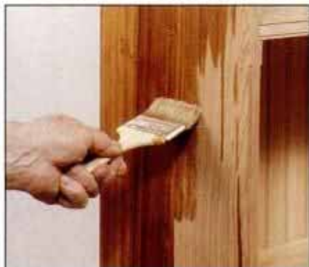
19 Apply wood conditioner before staining to prevent blotchy, uneven coloration. Wipe off excess after 10 minutes.
