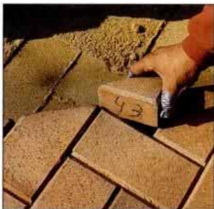
17 Fit all cut pieces back into the pattern following the numbers. If a piece is a little too long, recut it.
