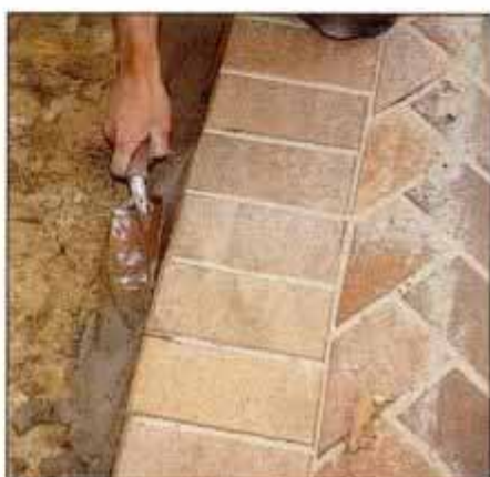
21 Dig a 4-in.-wide \times 6-in.-deep trench where the bricks meet the soil. Fill with concrete to keep the bricks from moving.
