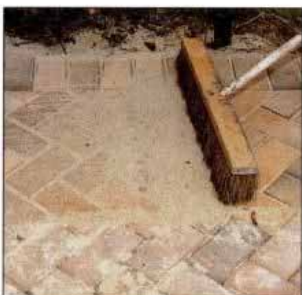
20 Once all the cracks are filled with sand, sweep up any extra sand and rinse the entire surface with water.
