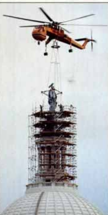
Four cables run from Skycrane to a lifting ring in the statue's base.
