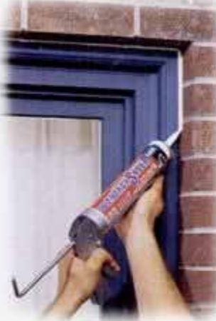
USE IT AROUND DOOR JAMS, AROUND WINDOW FRAMES. ANYWHERE YOUR HOME LOSES ENERGY.
