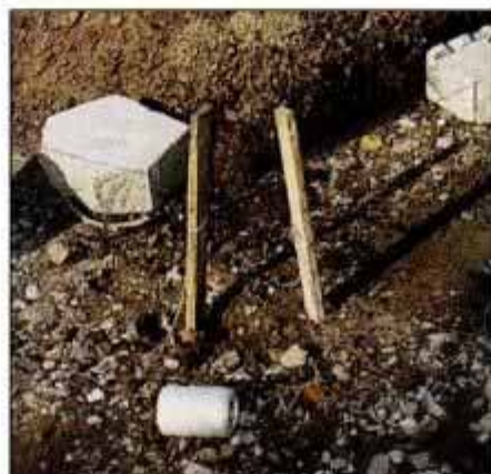
5 If you need a retaining wall, like we did, lay out the position of the wall using level mason's string, as shown.
