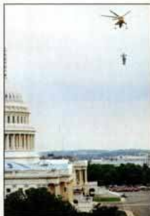
Four cables run from Skycrane to a lifting ring in the statue's base.
