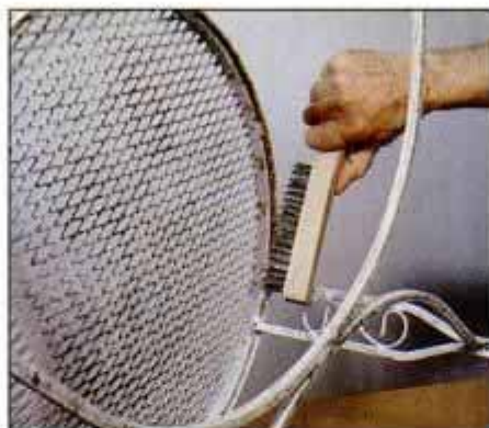
4 Use a hand wire brush to remove light rust from confined areas, such as the inside rim of a metal chair.
