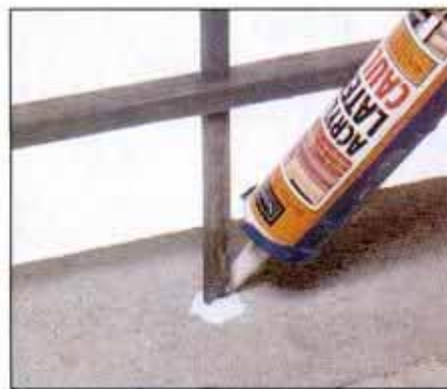
9 Seal a handrailing's post with a flexible exterior-grade caulk, such as silicone or acrylic latex.
