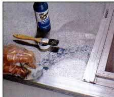
11 Remove corrosion on aluminum using Aluminum Jelly and a rag or plastic pad. Don't use steel wool on aluminum.
