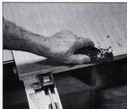
23 Glue edge banding to the plywood. Banding is slightly thicker than plywood and is planed flush after glue sets.
