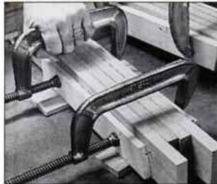
2 Use alignment nails to prevent the two pieces of the top rail from sliding while you are gluing and clamping them.
