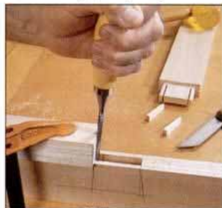
15 Cut a tapered mortise of a fox-wedged joint with a chisel and guide block. Make mortise 1/8 in. deeper than the tenon.
