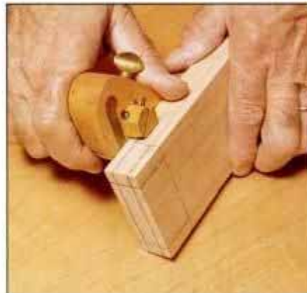
2 Use a marking gauge to lay out the tenon cheeks and sides of the mortise. Scribe shoulders with a knife and square.
