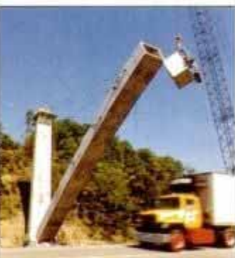
Cables hold segments of Natchez Trace Arches in place until each complete arch is created.
