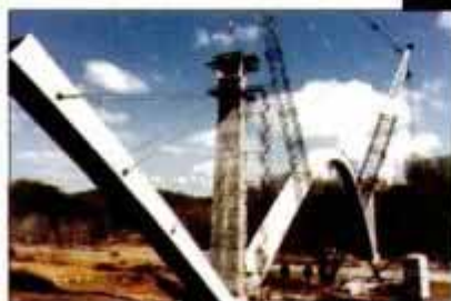
Cables hold segments of Natchez Trace Arches in place until each complete arch is created.
