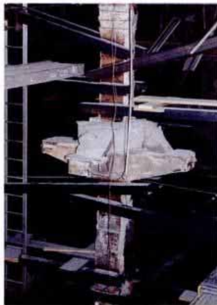
Above, new steel tubes brace vertical column, shorn of its supporting concrete floor slabs by the blast.
