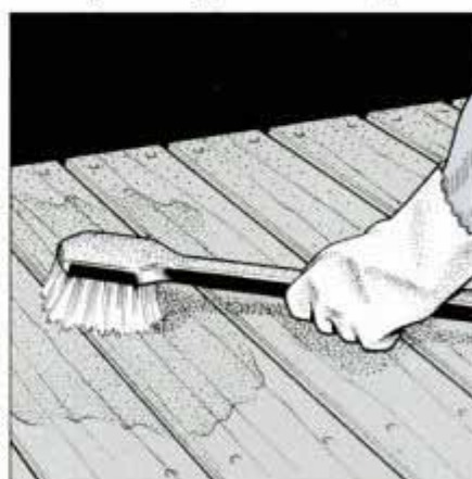
2 Apply a deck brightener with a stiff brush to remove stains and weathering. Follow manufacturer's instructions.
