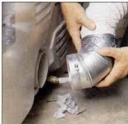
21 Remove the dryer's vent tube twice a year and shake or vacuum out the accumulated lint and debris inside it.
