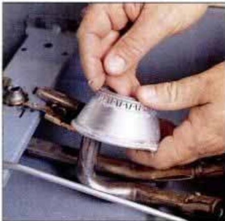
8 Gently clean soot from the burner openings using a safety pin. Work around the burner's circumference.
