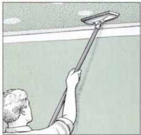
14 Smooth the compound with fine sandpaper and use a sanding stick to easily handle hard-to-reach areas.
