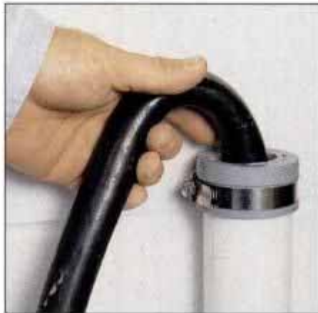
19 Install a rubber friction fitting to firmly fasten the washer discharge hose inside the plumbing standpipe.
