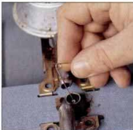
6 Clean soot and carbon from the pilot orifice using a safety pin. Work gently to avoid damaging the orifice.
