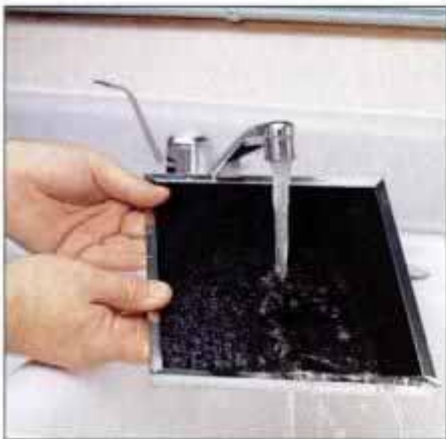
11 Rinse dust and grease out of the hood filter using hot water. Let the filter dry before reinstalling it.
