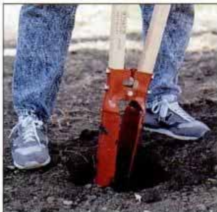
1 A scissors-type post-hole digger works well in digging deep narrow holes and squaring the hole bottoms.
