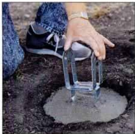
4 A post bracket has tabs that penetrate the concrete. Press brackets in place so the tabs are fully embedded in surface.
