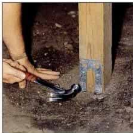
6 When fastening support posts to the footing bracket, use approved bracket nails for maximum joint strength.
