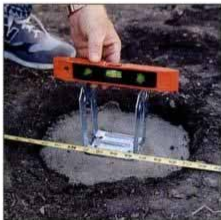
5 Use a tape measure or taut string to determine the exact bracket position. Then, level the bracket in both directions.
