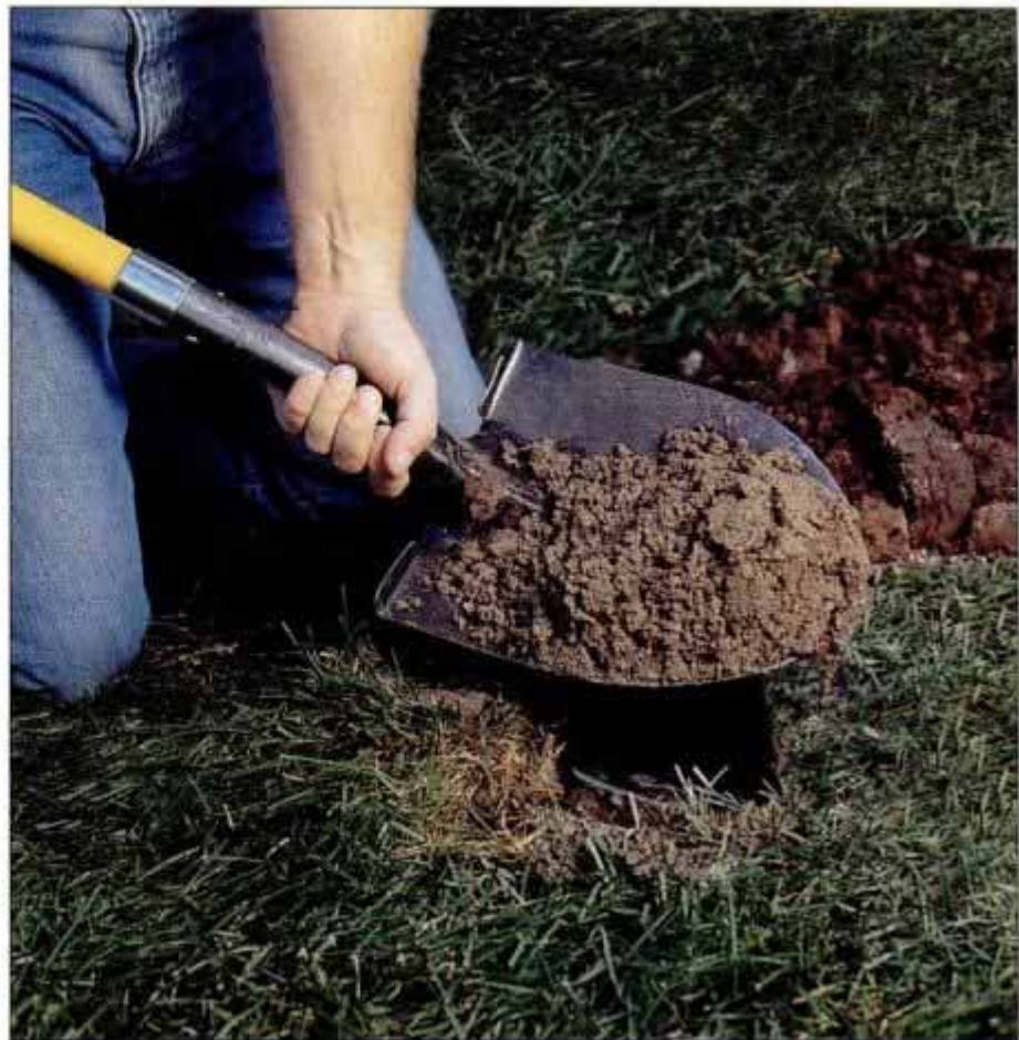
A concrete footing set below the frost line provides a stable base for deck and porch construction. Premixed concrete is the easiest solution for small jobs.
