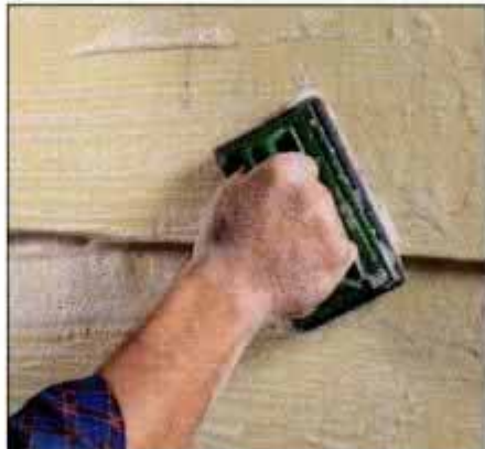
2 Rinse the siding with water first, then scrub the surface with a mild household detergent and stiff cleaning pad.
