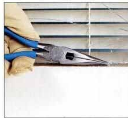
2 Once the putty is out, find the glazer's points and remove them with needle-nose pliers or a screwdriver.
