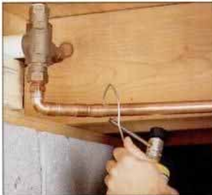
8 Join the supply tubing to the valve with lead-free solder. Protect any nearby framing members with sheetmetal.
