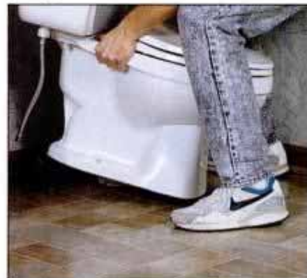
2 New vinyl flooring should be installed under, not around, a toilet. Remove the toilet and reset it later.
