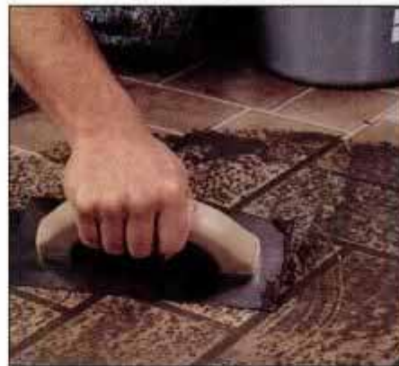
10 To smooth out embossed flooring, apply leveler to the surface. Once recesses are filled, scrape away excess.
