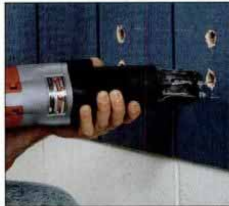
3 Use a reciprocating saw, or a sabre saw, to cut between the holes. Working slowly will yield the straightest cut.
