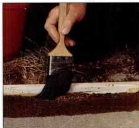
4 Thoroughly remove any debris from the damaged area. Make sure to dampen the surface with water prior to patching.
