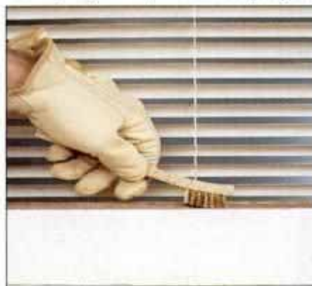
4 Use a wire brush or a sharp chisel to clean off the sash. Wipe away loose particles before installing a new pane.
