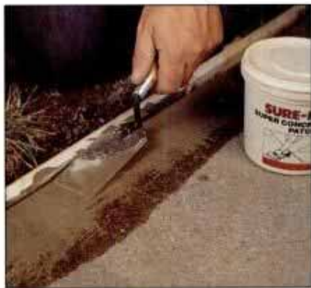
5 Apply the patching material to the crack using a small trowel. Feather the patch to match the surrounding surface.
