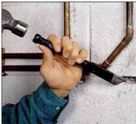
6 Remove loose or cracked mortar between blocks with a tapered mason's chisel, and clean the joint thoroughly.
