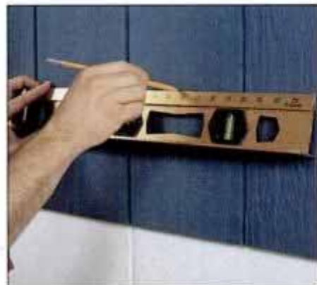
1 Position the faucet in a convenient location, then mark the siding for the faucet body cutout using a level.
