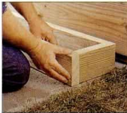
13 Preassemble a box step using the drawing as a guide. Set it on a poured concrete pad or a few concrete blocks.
