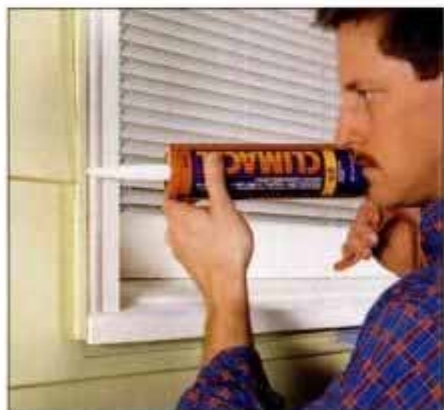
3 Use silicone caulk to seal all joints where the wood and siding meet. Pay special attention to windows and doors.
