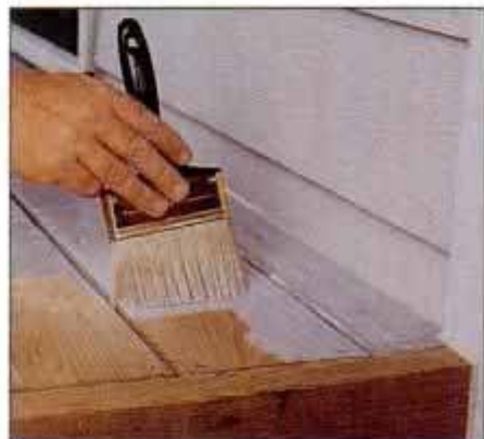
17 After sanding away any rough spots and removing the dust, cover the deck with wood sealer or an oil-base stain.
