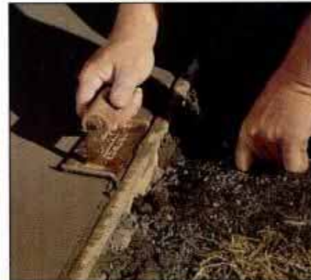
9 Use an edging tool to round off all edges. Then gently retrowel the surface and brush lightly with a broom.
