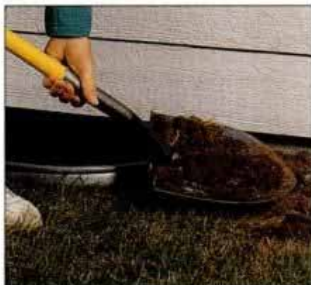
2 Add soil to any depressions around your foundation. Then tamp the soil firmly into place and plant grass seed.
