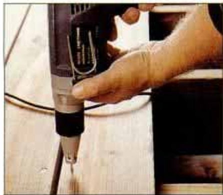
12 Drive the deck screws with a standard drill or a screw gun like we did. Set screws just below the surface.
