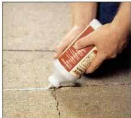
1 Brush away debris from any cracks, then pour in liquid-polymer crack filler to a level just below the surface.
