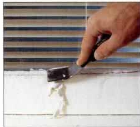
8 Smooth the putty by drawing a clean knife firmly along the joint. Carefully trim away any excess when finished.
