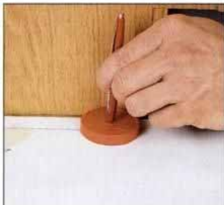
7 To scribe the exact perimeter of the floor, insert the ballpoint pen into the roller disc and trace around the room.
