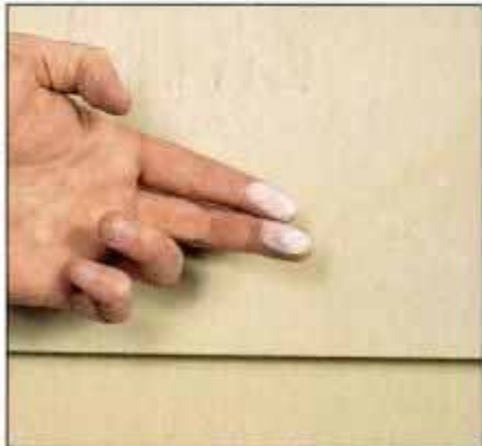
1 Wipe your fingers across the siding to check for chalking. If heavy dust comes off on your fingertips, consider painting.
