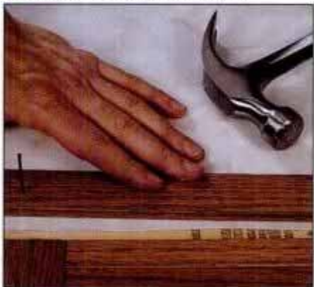
15 When laying vinyl next to hardwood flooring, buy a hardwood reducing strip and glue or nail it in place.
