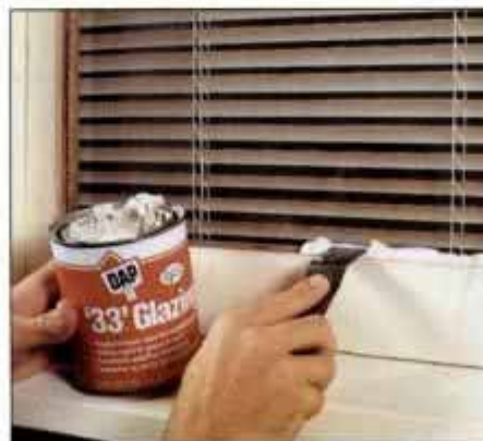
7 Install the glazer's points and then start filling around the pane with compound. Soften the putty before using it.
