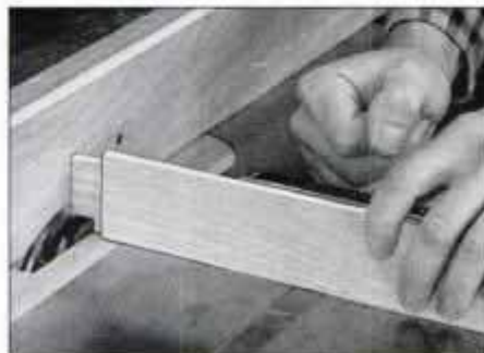
20 Tip the rails on edge, butt them against the fence and cut the shoulder on each upper door rail tenon.
