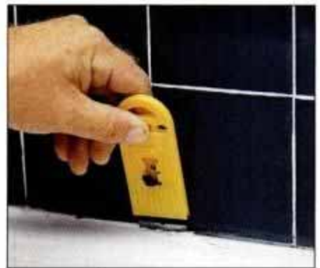
2 Use a razor-type scraper or sharp knife to cut away damaged caulk from around the tub. Then, clean the joints thoroughly.
