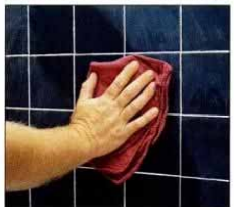
5 Rinse the cleaning solution with clean water and allow the surface to dry. Then, buff away the residue with a soft cloth.
