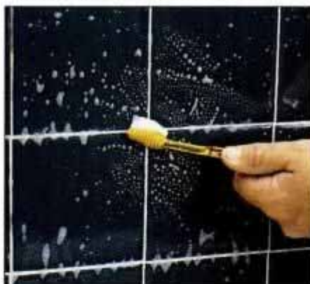
4 Stubborn stains can be removed with a toothbrush. Use a tile cleanser or ordinary household bleach diluted with water.
