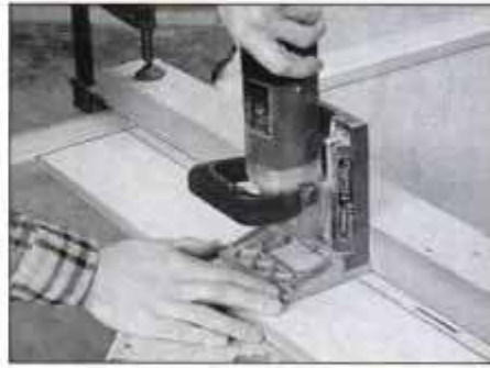
8 Cut joining plate slots on the back of the face frame using a straightedge to guide the plate joiner.
