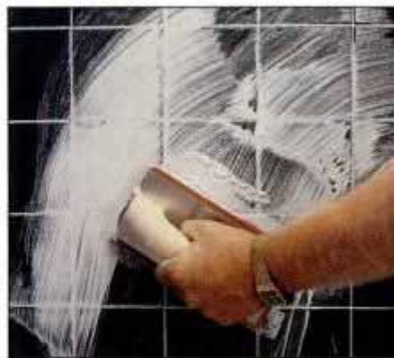
7 Use a rubber float to apply grout. Force grout into the joints between the tiles and then squeegee away the excess.
