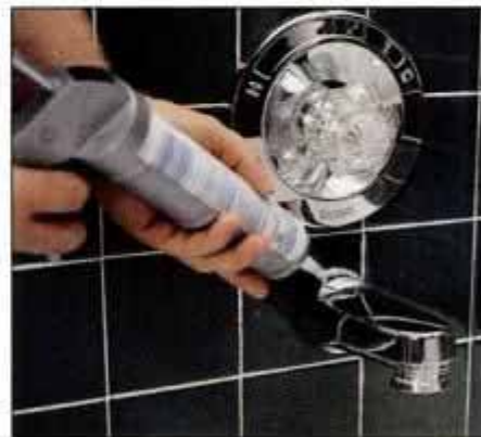
12 Apply a thin bead of caulk between the tub spout and tiled wall. Then, wipe away excess with a facial tissue.
