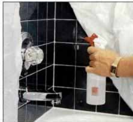
9 To slow drying by wet curing, drape plastic sheeting over tiles and coat the tiles with a mist of water several times a day.
