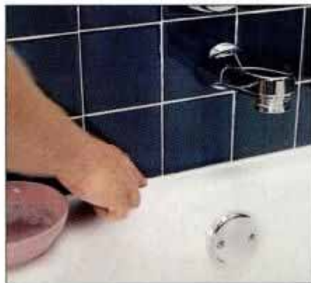
11 Smooth the caulk so it blends with the surfaces. Periodically wet your finger with soapy water to keep caulk from dragging.
