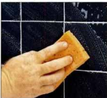
3 Use a tub-and-tile cleaner or homemade solution to remove soap scum, mildew or hard-water stains from tile.
