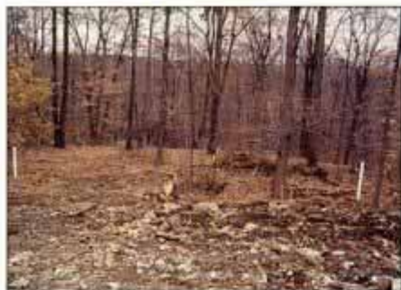
DAY 1. Project starts with 2-acre, pie-shaped, downward-sloping lot. White perk test pipes help determine septic location.
