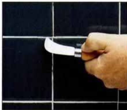
1 Use a carpet knife or grout-removal tool to clear loose grout. Remove grout a few inches to either side of affected area.
