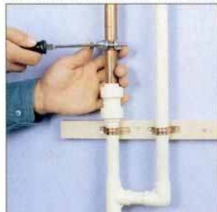
18 To reestablish an interrupted ground, secure an approved clamp to the metallic pipe on each side of the plastic pipe.
