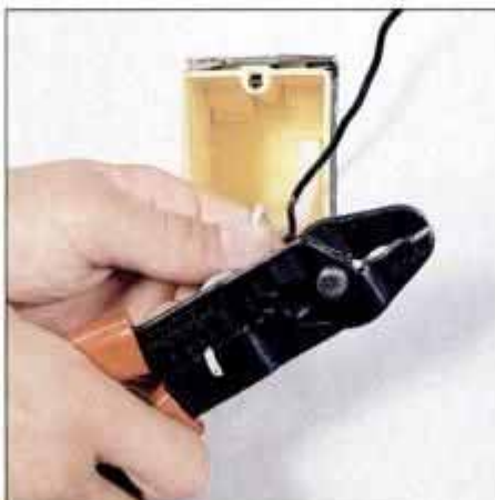
12 Strip roughly \frac{1}{2} in. of insulation from the ends of each switch loop wire. A wire-stripping tool best handles the job.
