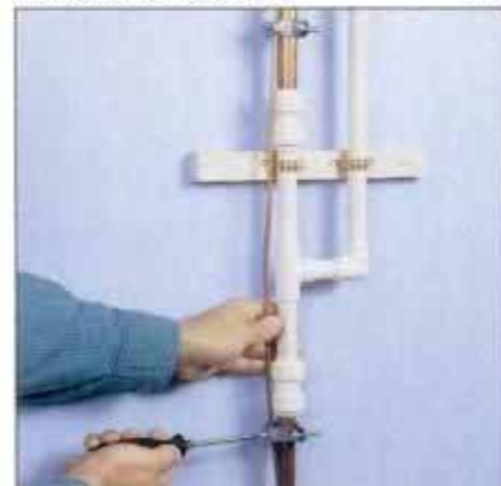
19 Connect the two grounding clamps with a length of No. 4 ground wire. Tighten the fastening screws securely.
