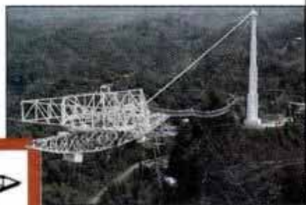
Dome (left), as big as a 5-story building, will replace existing antennas (right) on platform suspended over Arecibo's 1000-ft.-wide reflector dish.
