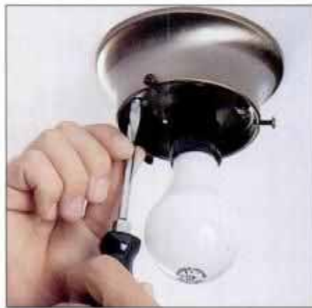
6 Loosen the screws that secure the fixture base to the ceiling box. Then, carefully pull the fixture down from the ceiling.
