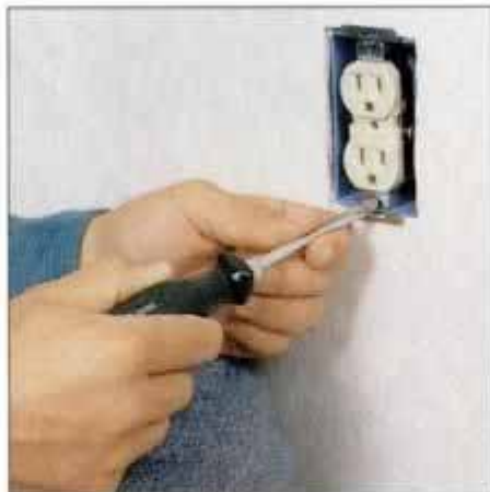
14 Remove a defective receptacle just as you would a switch. Take off the cover plate and remove the switch yoke screws.
