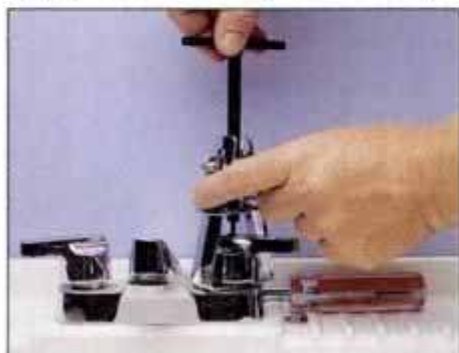
27 If you can't remove a faucet handle by gentle prying with a screwdriver, use a handle puller to free the stuck handle.
