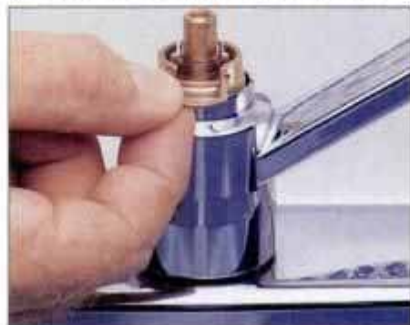
32 To free the valve cartridge from its housing on this single-faucet unit, pull the small, U-shaped brass key from its slot.
