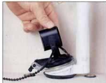
18 Press the new seat and flapper onto the epoxy putty, connect the chain and wait at least 15 minutes for epoxy to set.
