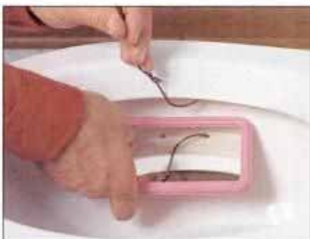
14 Use a coat hanger and hand mirror to clear bowl rim holes. Then flush and check for a good water flow down sides of bowl.
