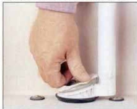
17 If flush valve seat is severely pitted, install flush valve kit with new seat. First, press epoxy onto worn flush valve seat.
