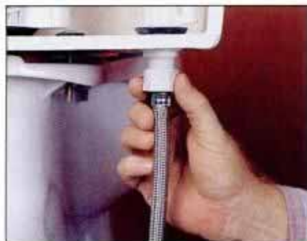
19 To replace a fill valve (ballcock), first remove all water from tank. Then, disconnect the fill valve supply tube nut.
