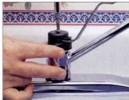
30 To access the cartridge on this Moen faucet, take off the hood, remove the handle screw and tip handle back to free it.
