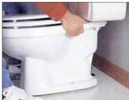
9 Lift the toilet by grasping the bowl only. Holding the tank can damage the seal between the bowl and the tank.
