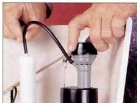
24 Feed the plastic fill-tube hose into the overflow tube and reconnect the tank water supply tube. Then, turn on water.
