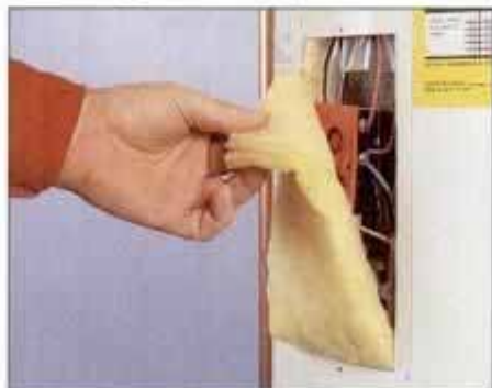
2 Remove the insulation under the panel cover. But, be sure to replace it so thermostat reads tank temperature accurately.
