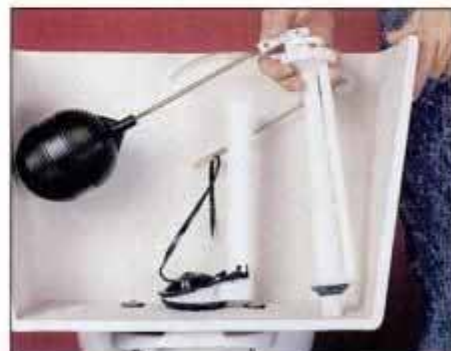
21 Finally, remove the old fill valve by disconnecting the fill tube and lifting the old assembly up and out of the tank.
