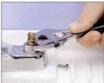
28 Once the handle is removed, use an adjustable wrench to loosen the bonnet nut that secures the valve stem.
