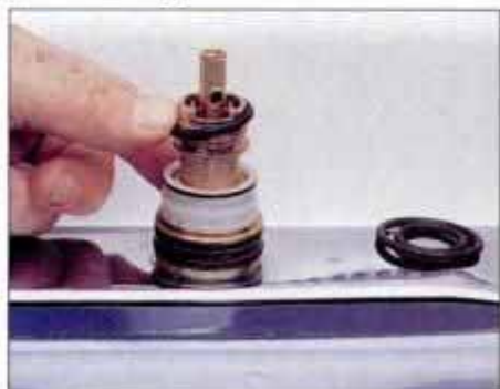
36 Grease the new O rings and roll them over the column until they seat themselves. Then, reassemble the faucet.
