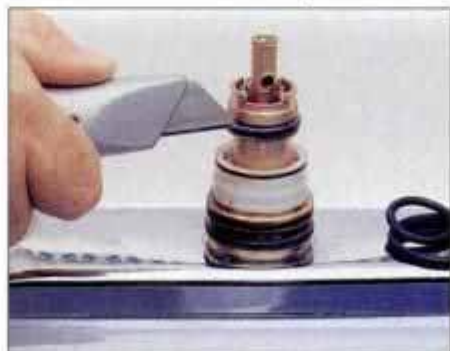
35 With new, appropriate O rings on hand, use a sharp utility knife to cut the old O rings from the faucet riser column.
