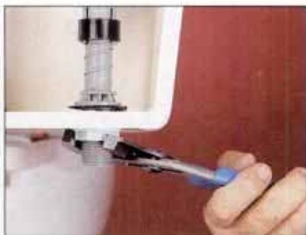
23 Tighten the new fill valve's jamb nut to lock the valve in place. If the jamb nut is round, use pliers to tighten it.
