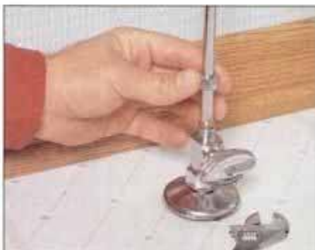
13 Reconnect the water supply tube by inserting it into the stop and tightening the compression nut.
