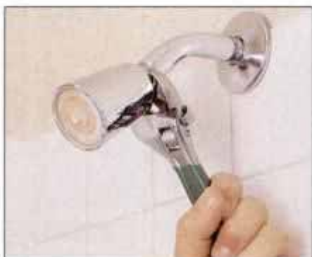
25 To clear a clogged shower head of mineral deposits, unthread the shower head from the arm with an adjustable wrench.
