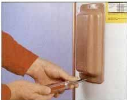
1 To change the temperature setting on an electric heater, first remove the panel covers to access the thermostats.
