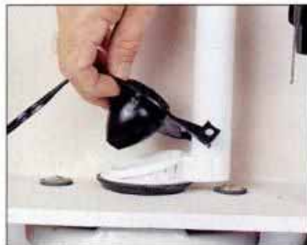
15 If a bad seal causes tank water to leak into the bowl, replace flapper valve with new valve attached to flush-valve pegs.
