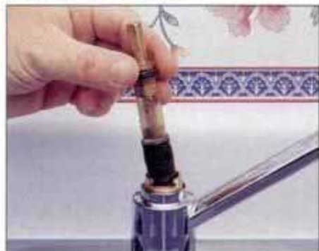
33 Simply lift out the old cartridge and install a compatible replacement. Lock the new cartridge in place with the brass key.
