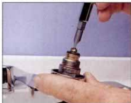
29 To replace a worn compression washer, undo washer screw, slide off old washer and install a new one of the same type.
