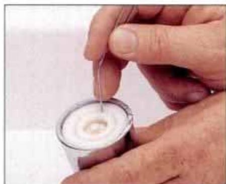
26 Soak the shower head in hot vinegar for 15 minutes to soften the deposits. Then use a paper clip to clear the openings.
