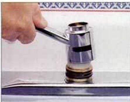
34 To remove the spout when replacing O rings, lift up firmly and twist the spout to release it from the faucet.
