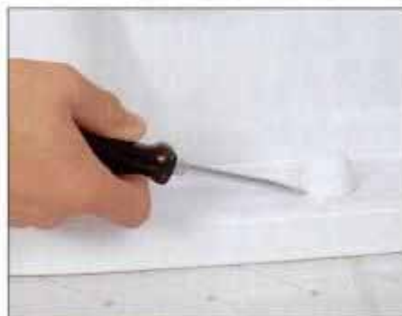
7 Use a screwdriver to pry up the decorative caps that cover the closet bolts on each side of the toilet base.
