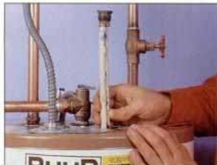
5 Lift the old anode rod from the heater, then slide in the new rod. Apply a light coating of joint compound to threads.
