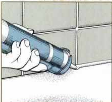
2 Hold tube at 45° angle to run bead along joint. Use gentle trigger pressure and progress slowly. Then, turn plunger rod so notches face up to reduce excess caulk flow.
