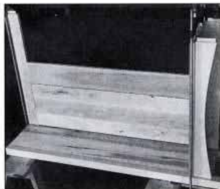
18 Glue and clamp the back rails and mullion. When the glue is dry, slide in a back panel. Clamp this to a side.
