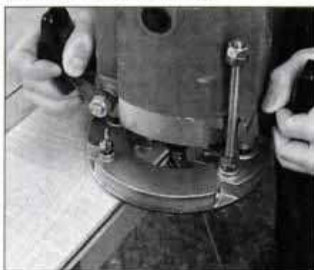
13 Secure the mullion to the workbench and use a slotting cutter to cut the groove that holds the back panels.
