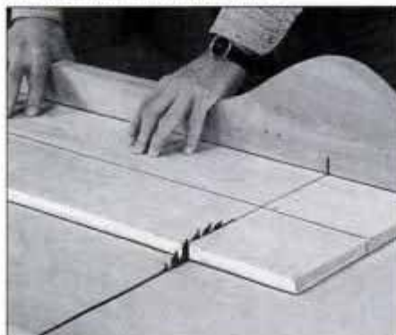
3 Use a sliding crosscut table on the table saw, or a circular saw and guide, to cut the panels to length.
