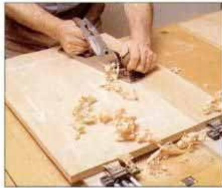
12 Apply glue to slots, plates and mating edges, then clamp. When dry, smooth panel surface with hand plane.
