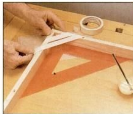
7 Fabricate the apron pieces, then join them with glue and brads. Hold the joint in square alignment using masking tape.
