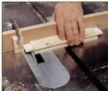
10 Use a dado head in a table saw to cut the tenons on the ends of the door rails.
