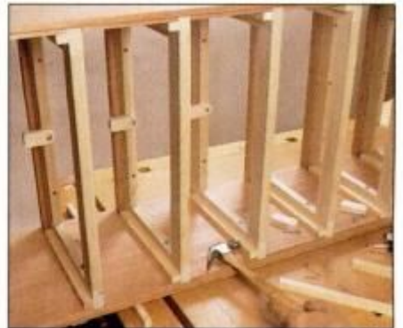
15 Cut drawer spacer cleats to size, then nail them to bottom edge of frame members, not to the case side.
