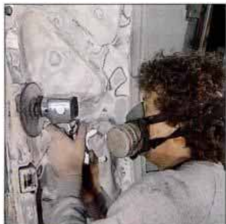
Ken Barnes uses a DA sander on the inside of the trunklid prior to priming and painting.
