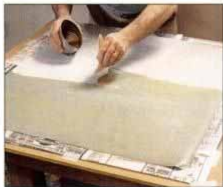
12 Cut the sheet vinyl to rough size. Then using a short bristle brush, apply contact cement to its bottom side.
