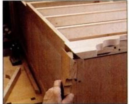
20 Cut case feet to shape and join to mounting cleat. Then glue and screw to bottom, using plate to reinforce corner.
