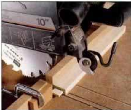
6 Cut to size narrow stock that closes front of the dados. Use plate joiner to cut matching slots in side and strip.
