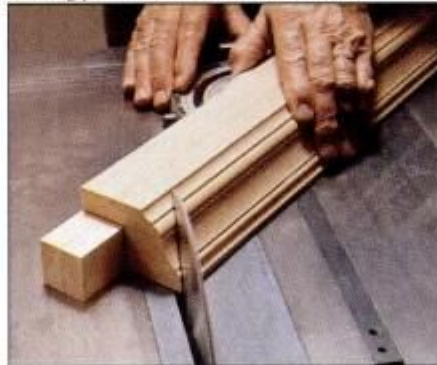
19 Join crown molding parts with glue and screws. Then support back side of assembly with scrap block. Cut miters.
