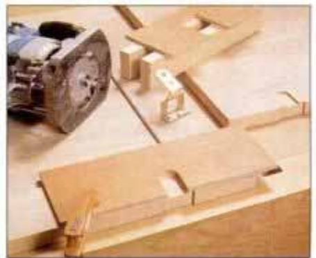
16 Cut hinge mortises using router with guide bushing and two scrap wood jigs—one for door surface, one for door edge.
