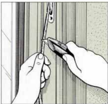
3 If the sash cords are still in place, cut them off with a utility knife and let the sash weight pull them through.
