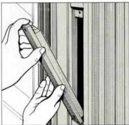
4 Back out the screw or nail at the top of the sash-weight door, then remove the door. Take out the sash weights.
