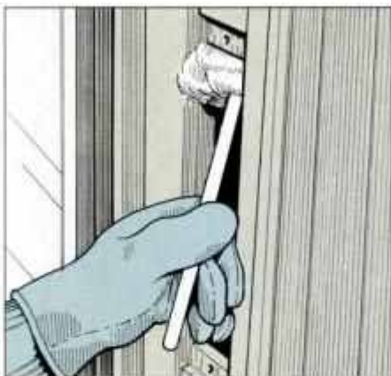
6 Stuff fiberglass insulation into the jamb weight cavity. Tear the insulation into pieces, and use a pushstick.
