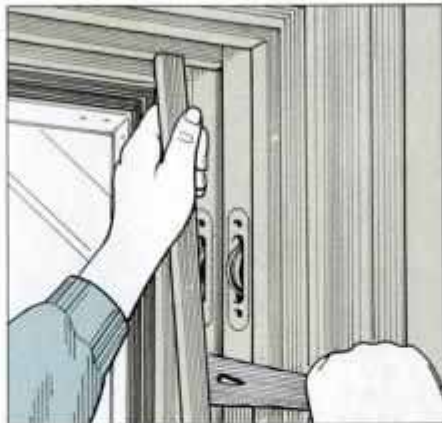
2 The parting stop holds the outside sash in place. Remove it by prying it out of the slot in the jamb or chisel it flush.
