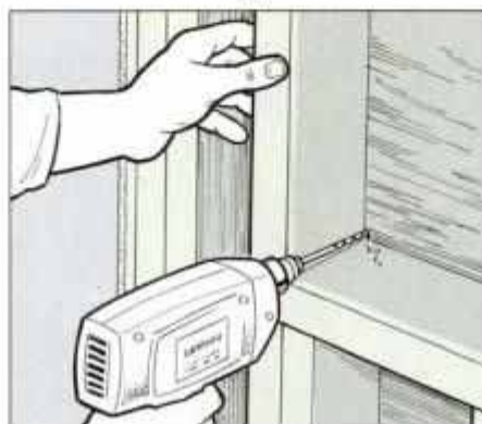
16 To mark the location on the outside of the house, bore through the sheathing and siding at each corner of the opening.
