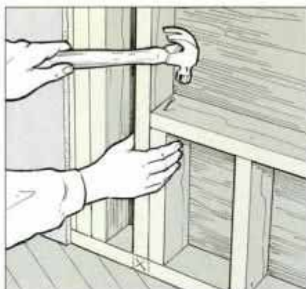
13 Toenail the sill into the vertical studs, and nail directly through the face of the sill, into the end of the cripples.
