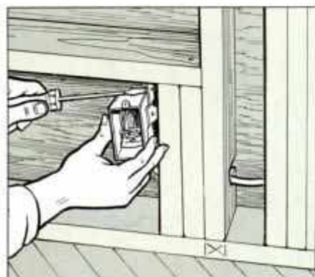
15 Position the electrical box right below the sill, and screw or nail the box to the cripple studs.
