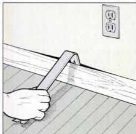
1 Pry baseboard off the wall and remove outlet covers. You may see stud markings on wall framing behind baseboard.
