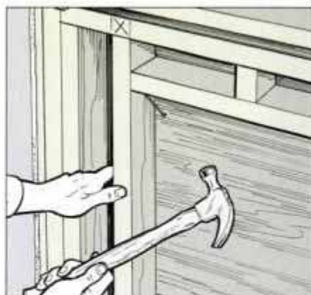
14 Before installing the header, start toenails at corners. Nail the header to the cripples above it, then drive in toenails.
