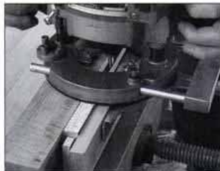
8 Cut the mortise in the rear rail with a plunge router. To support the router's base, clamp a block next to the rail.
