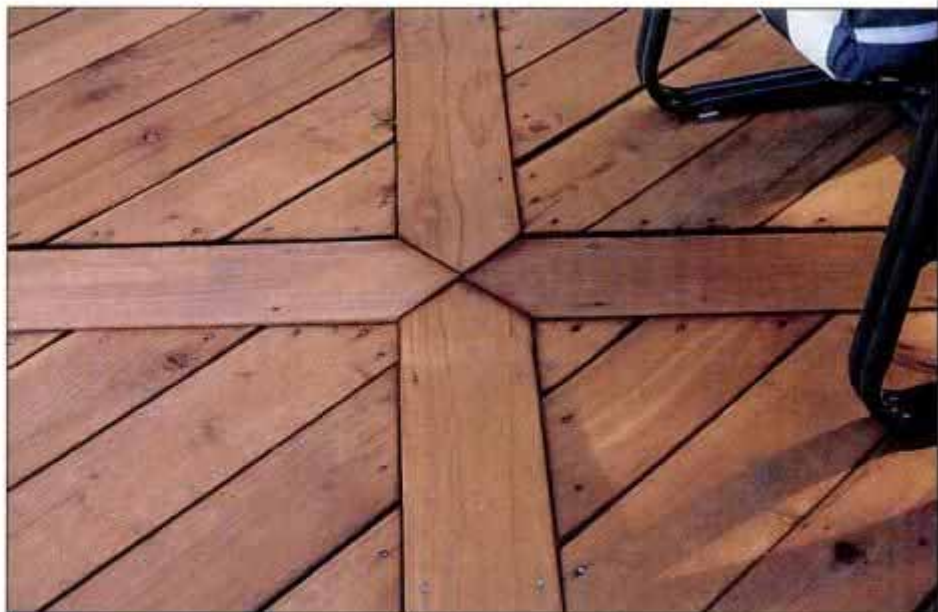
Tasteful design elements include belt boards that intersect at the middle of the main deck. The decking is laid diagonally, and the perimeter is trimmed with redwood.
