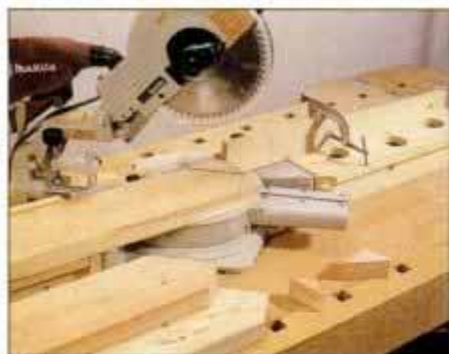
9 When cutting repetitive miters, such as rafter ends, use a stopblock clamped to the extension tables to locate each piece.
