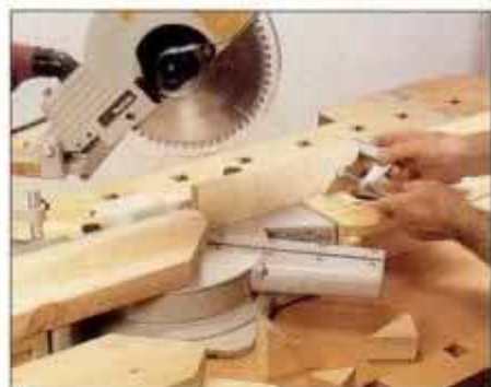
10 Make the bottom rafter cut by flipping over the rafter and aligning work with blade. Install stopblock and cut all rafters.
