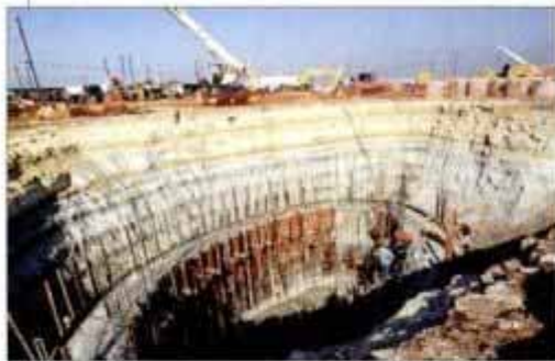
Magnet-delivery shaft is oval-shaped to accept magnet tubes, which can't be tilted.
