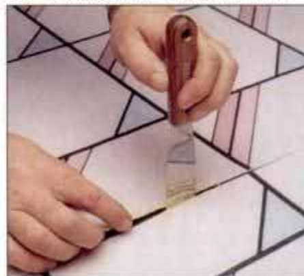
12 To repair a slightly separated seam, first apply mastic to the underside of both pieces of vinyl using a putty knife.
