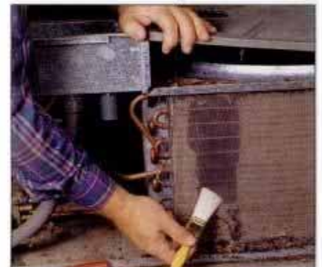
4 Remove the side panels on the condenser and use a soft brush to remove the dust that accumulates on the fin tubes.
