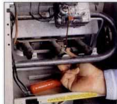
10 To adjust the burner, loosen the set-screw on the air-mixture mechanism and slide it open or closed. Retighten the screw.
