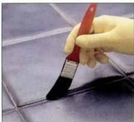
7 Ceramic tile floors do require periodic sealing. To do this, first apply sealer to all the grout joints with a stiff brush.
