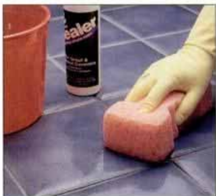
8 After the grout joints are sealed, apply sealer to the surface of the tile with a large sponge. Work with short, smooth strokes.
