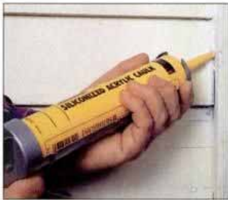
7 Once the primer has dried thoroughly, apply a new bead of caulk using flexible and paintable exterior-grade caulk.
