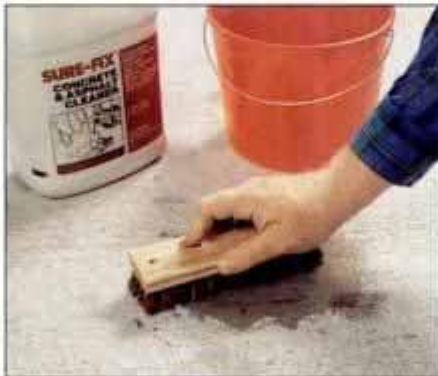
2 Remove stubborn oil stains with commercial degreaser. Brush area firmly to lift stain, then rinse off with clean water.
