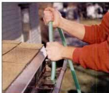
2 Remove stubborn clogs from downspouts using a garden hose to force a strong stream of water down the pipe.
