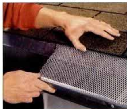
5 To install a full gutter screen, just roll out screening, cut it to length and force the top edge under the bottom shingle course.
