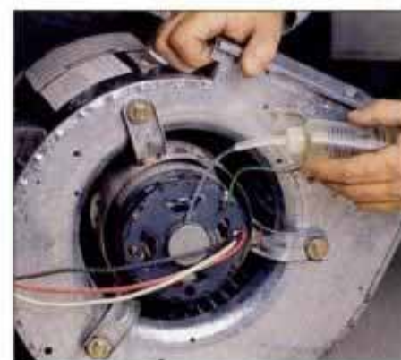
9 If your blower motor has oil ports, fill the ports on both sides of the shaft using an oil bottle with a long spout.
