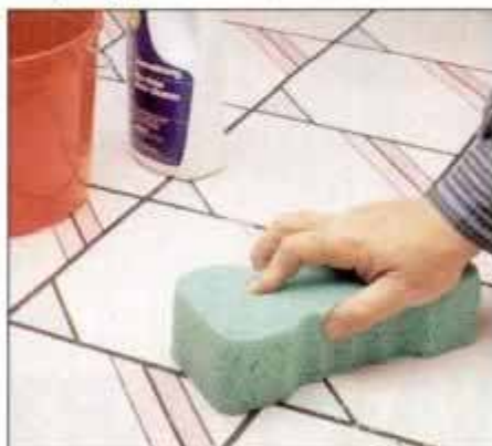
10 To clean vinyl flooring, scrub the surface with a sponge and no-rinse floor cleaner. Let the floor dry before using.
