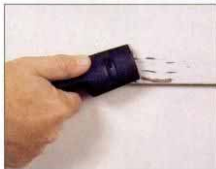
2 To touch up small peeled areas, first scrape away any curled or peeling paint. Use a scraper with replaceable blades.
