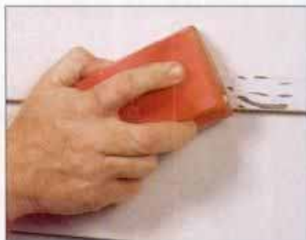
3 Once the scraping is done, sand the peeled paint edges to match the surface of exposed siding using medium-grit paper.
