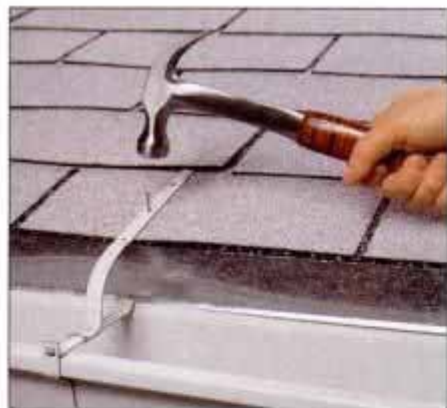
8 To lift a sagging gutter that is supported by brackets, remove the nails, reposition the brackets and nail in place.
