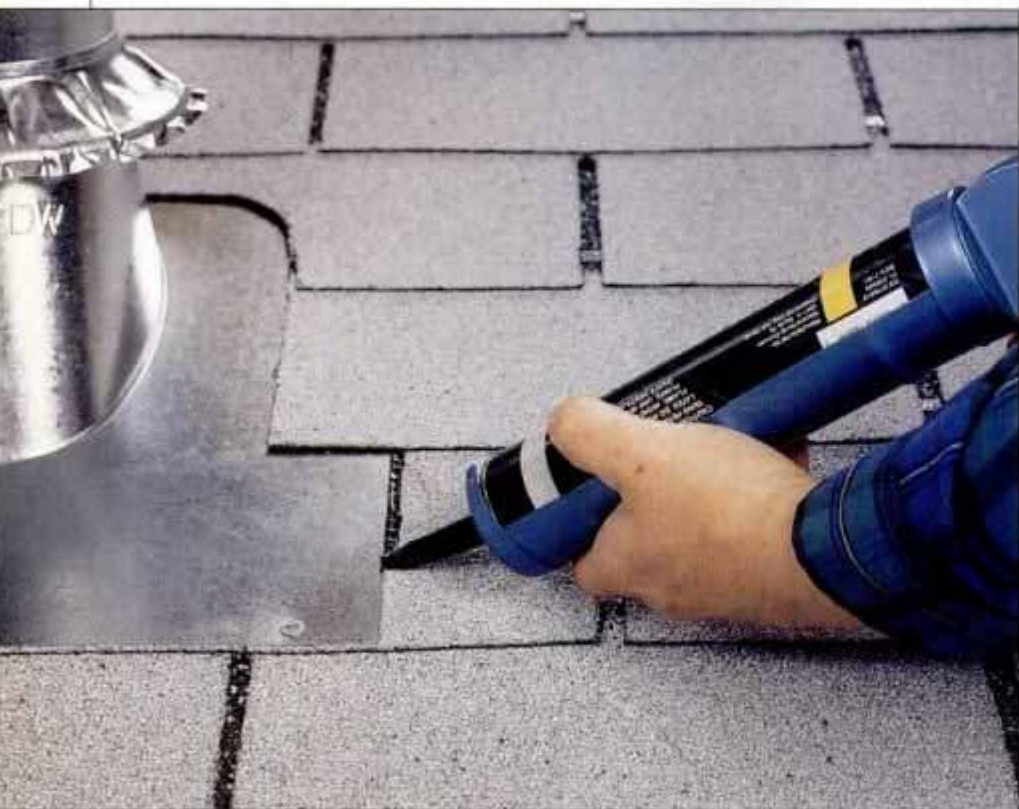
1 To properly seal flashing components that lie on top of surrounding shingles, apply a thick bead of roofing compound to bridge the joint between the two surfaces.
