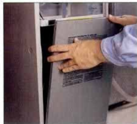
6 To access the furnace blower—and in most cases the unit filter—remove the lower panel on the front of the housing.
