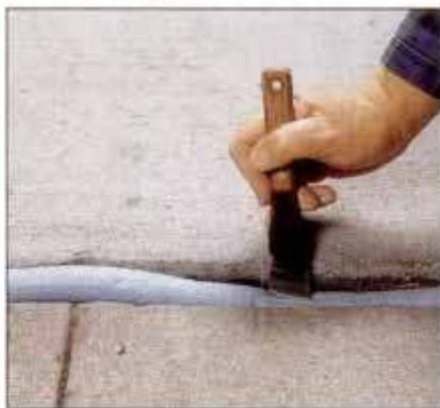
5 On particularly wide joints, it's a good idea to use flexible backing rod to fill the bulk of the void before caulking.
