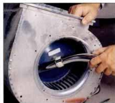
8 To thoroughly clean the blower unit, first remove it from the furnace housing, then vacuum clean the motor and fan.
