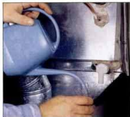
5 To keep the condensate drain on the evaporator free of bacteria, pour a mix of bleach and water through the hose.
