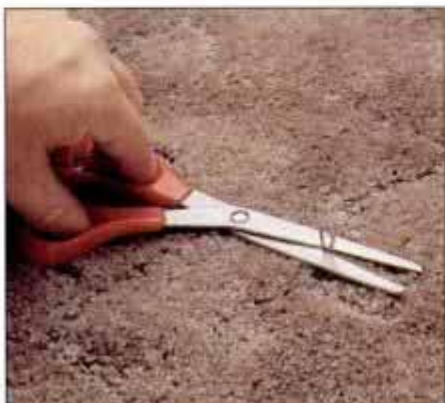
4 To prevent carpet snags from being caught again and again, trim off any pulled loops with a pair of scissors.
