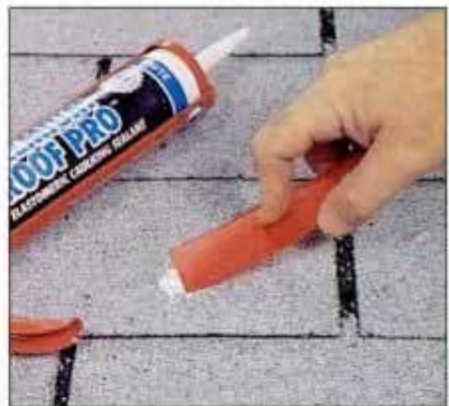
8 Smooth the compound in place using a putty knife. A light-colored compound works better with light shingles.
