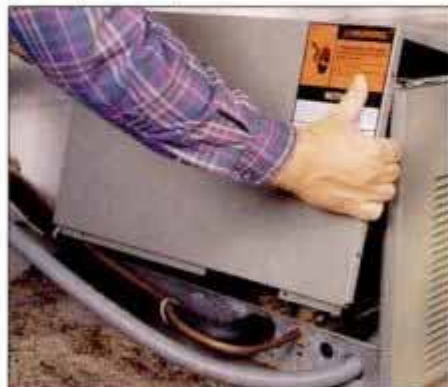
2 To gain access to the condenser unit, remove the front panel screws. Then lift the panel up and out to clear its bottom lip.
