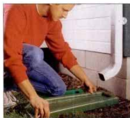
10 To help carry rainwater away from the foundation, be sure to install splash blocks under all the gutter downspouts.
