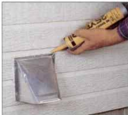
3 Because a dryer vent tends to span more than one course of siding, voids where the siding boards lap must be filled with caulk.
