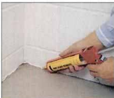
4 Caulk the cracks along basement walls and floors to keep insects from entering, or living in, these hospitable places.
