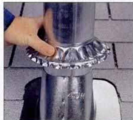
4 To properly seal a flue pipe, install a storm collar. Just slide it over the top of the pipe and down onto the flashing.
