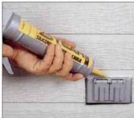
2 Exterior receptacles are another source of major air leaks. Caulk around the entire perimeter of the covering plate.
