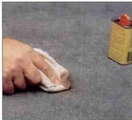
6 Repeatedly dab with the clean area of a solvent-dampened cloth. Rubbing the surface often results in smearing the stain.
