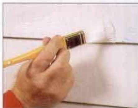
5 Once the primer has dried thoroughly, apply the topcoat with a touchup brush or similar narrow bristle brush.
