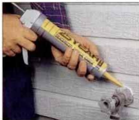
4 Silicone flanges rarely seat flush against siding. By caulking completely around the flange, air infiltration is eliminated.
