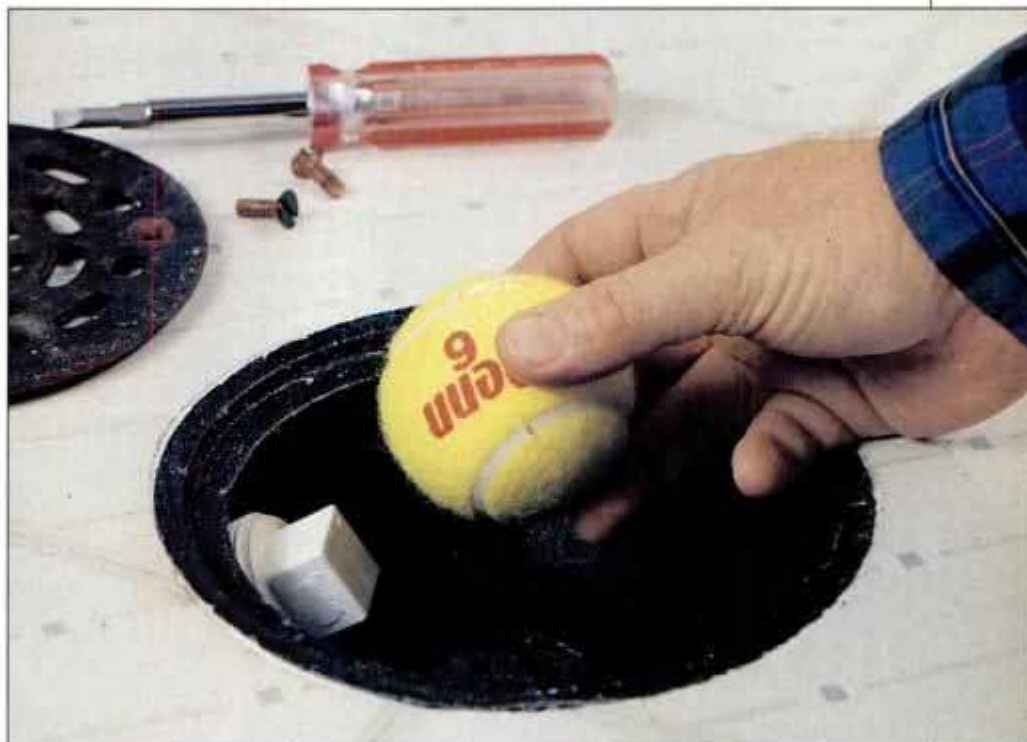
1 A basement floor drain can be a pathway into your house for various insects. A tennis ball placed in the drain can block the path and still allow water to pass.
