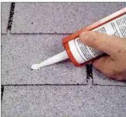
7 Fill the hole with elastomeric roofing compound. If it's more than 1/4 in. wide, put compound under the shingle, too.
