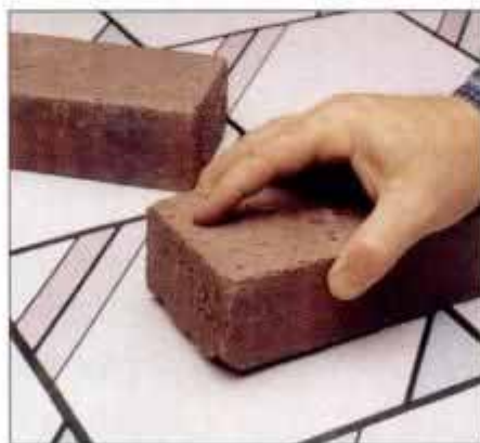
13 Hold the seam together by covering it with a brick or heavy book. Keep the weight in place for a day or two.
