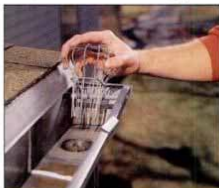
4 To keep debris from clogging downspout, insert a ball-shaped screen in top of spout. The screen just slides into place.
