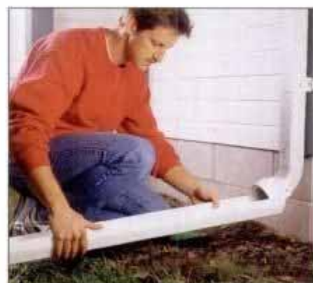
13 Once installed, the folding extension is easily lifted up and out of the way when you're mowing close to the house.
